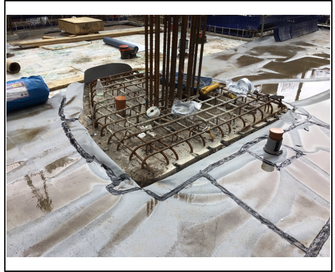
Overview of seal to pile cap
