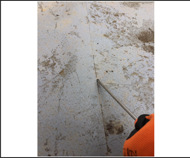
Pick and probe test carried out
