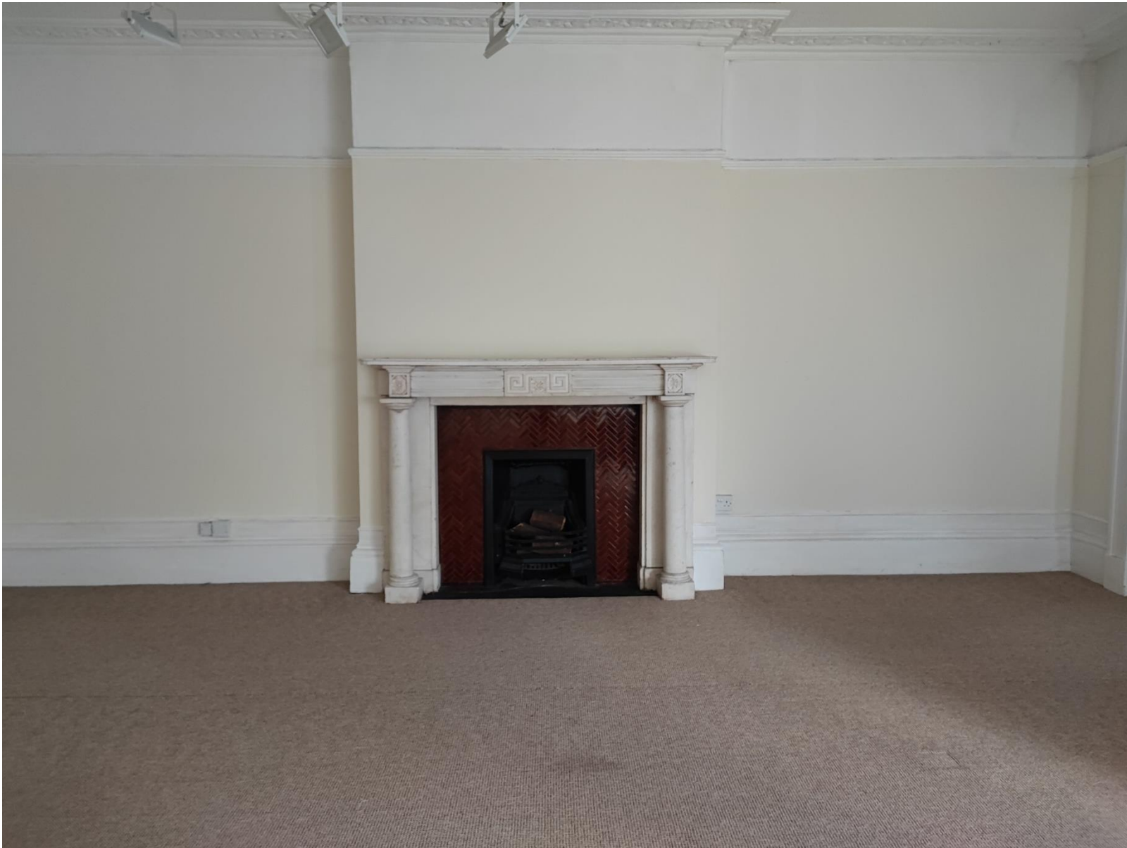
Figure 19 – View East towards the existing chimney breast fireplace from the front room. Installation of new partitions to the room.
