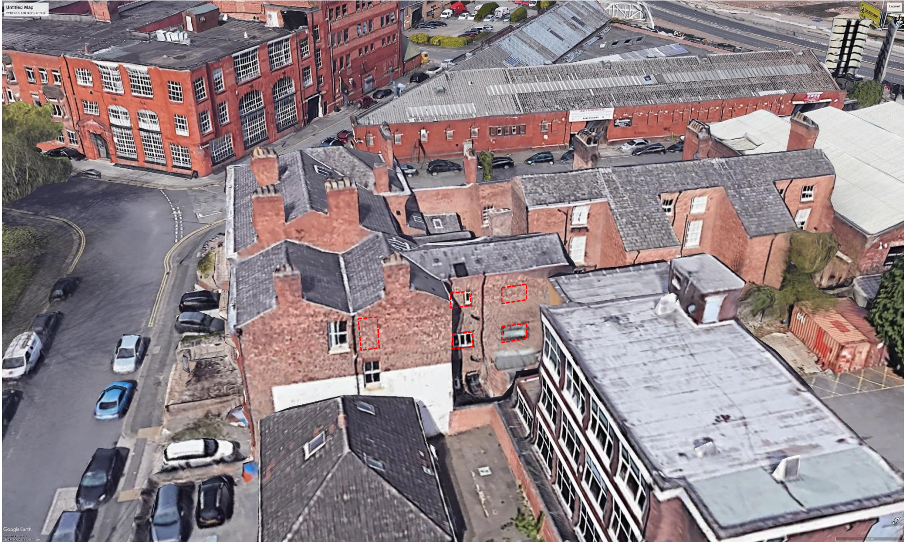
Figure 33 – Aerial view West towards the side elevation. Approximate locations for the new window / window enlargement dotted in red.
