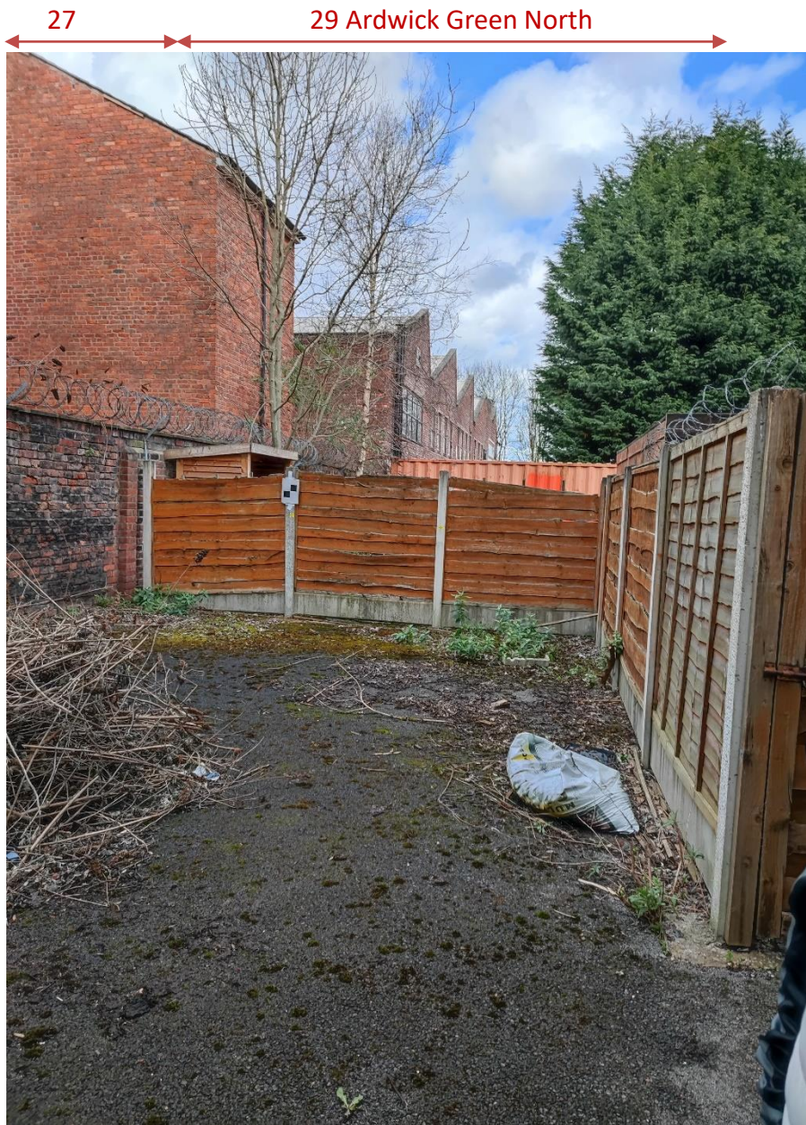
Figure 03 – View Northeast towards existing rear boundary treatment Timber fence to make good with a swing gate to the rear
