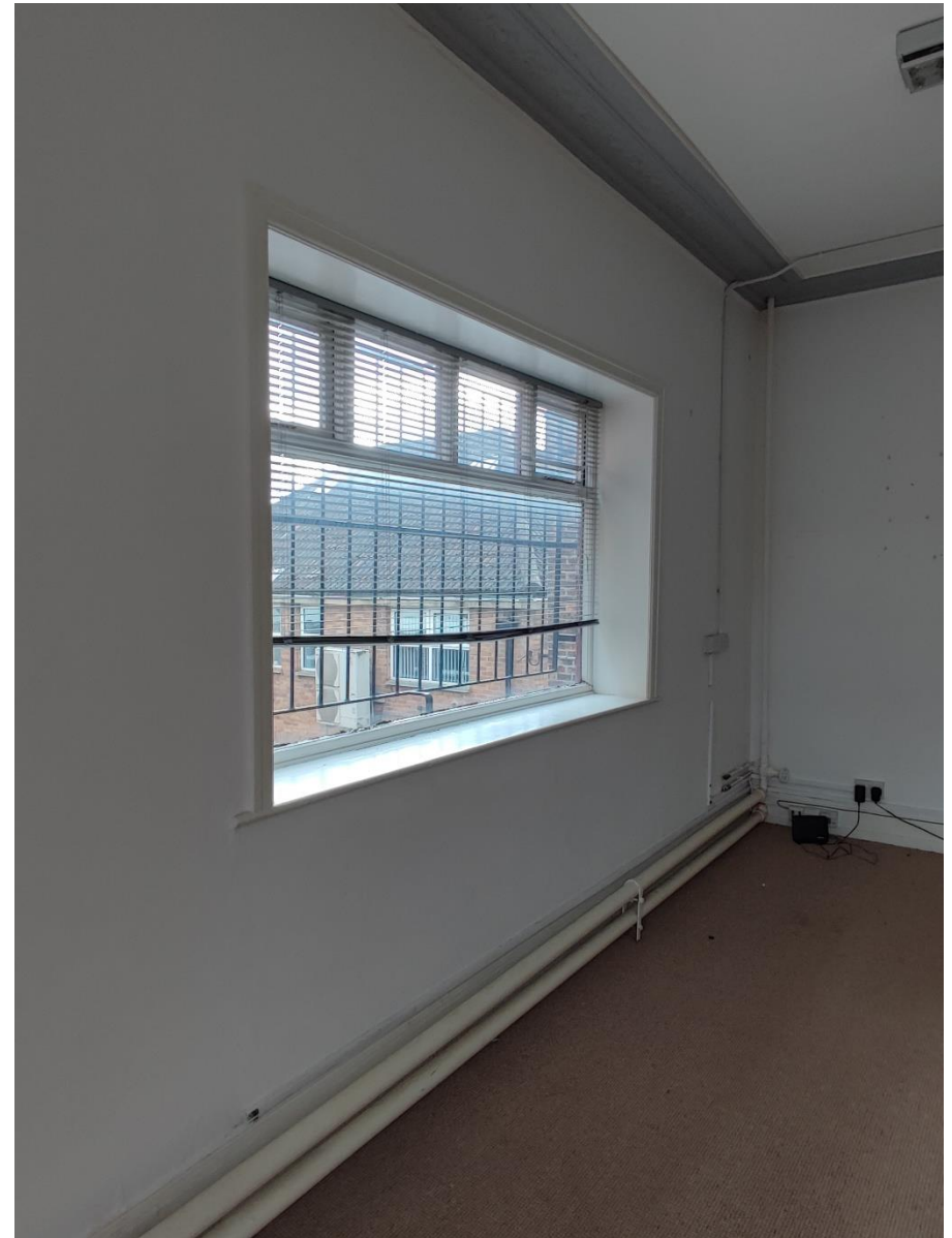
Figure 23 – View Southeast towards existing window from the rear room.
