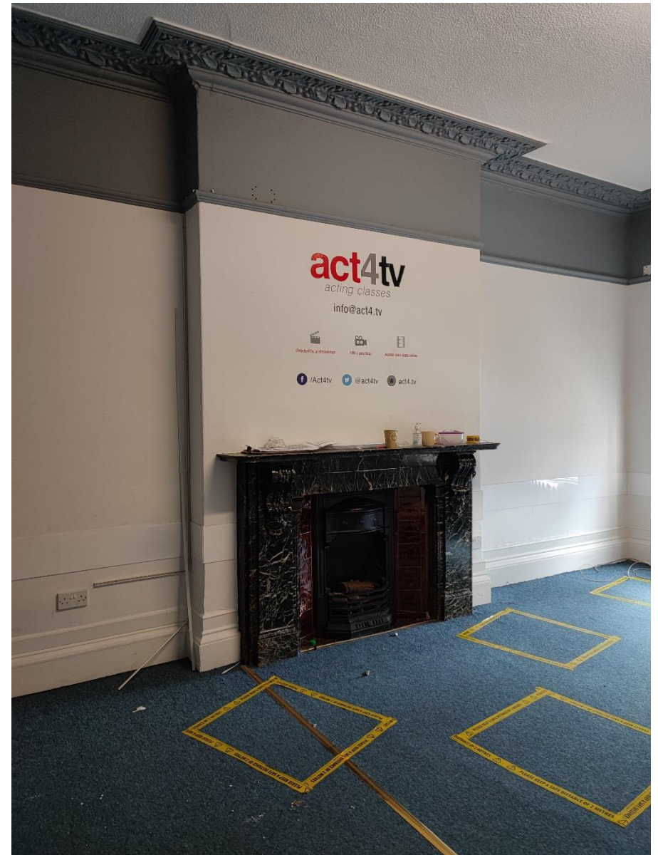
Figure 14 – View East towards the existing chimney breast fireplace from the front office. Existing fireplace to be covered.
