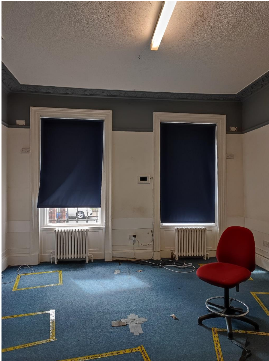
Figure 13 – View Southwest from the front office Installation of new partitions to the room.
