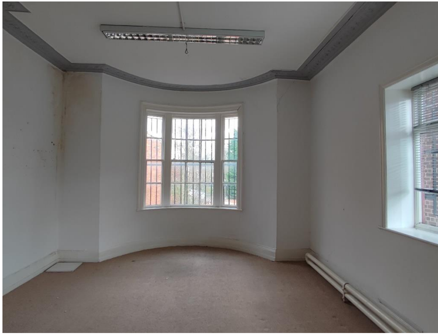
Figure 22 – View Northwest from the rear room. Installation of new partitions to the room.
