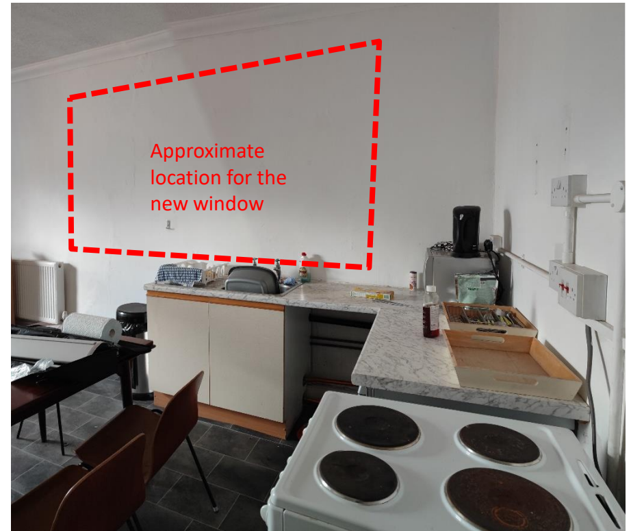
Figure 29 – View East from the rear room towards the side (East) elevation. Existing kitchenette to be removed, install a new window. Opening location and window style would be similar to the window on first floor, refer to Fig 23.
