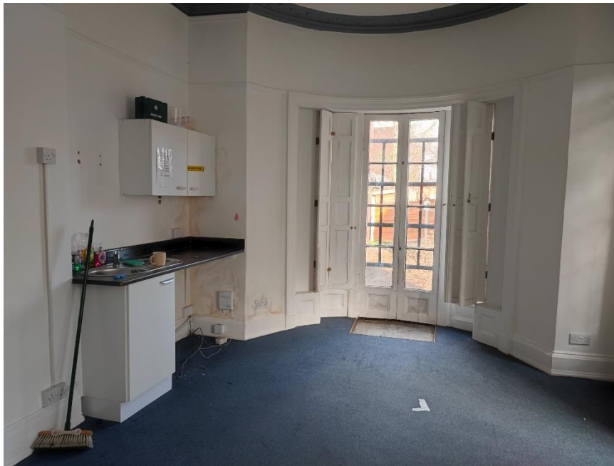
Figure 17– View Northeast towards rear yard from the rear office room. Existing kitchenette to be removed, install new partitions.
