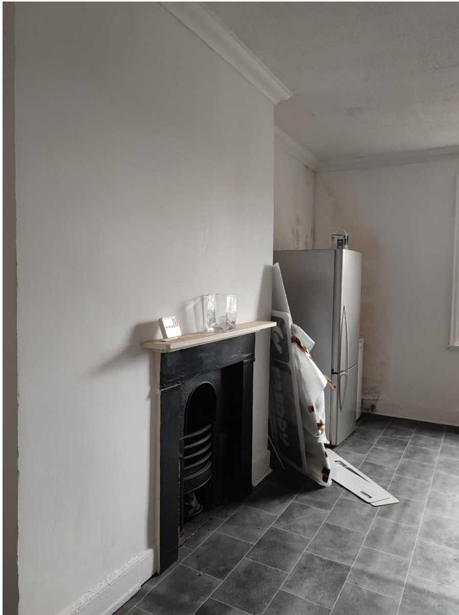
Figure 28 – View North from the rear towards the existing chimney breast fireplace . Fireplace to be covered.
