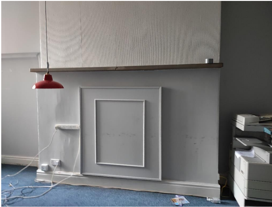
Figure 15– View East towards the chimney breast from the middle office room.
