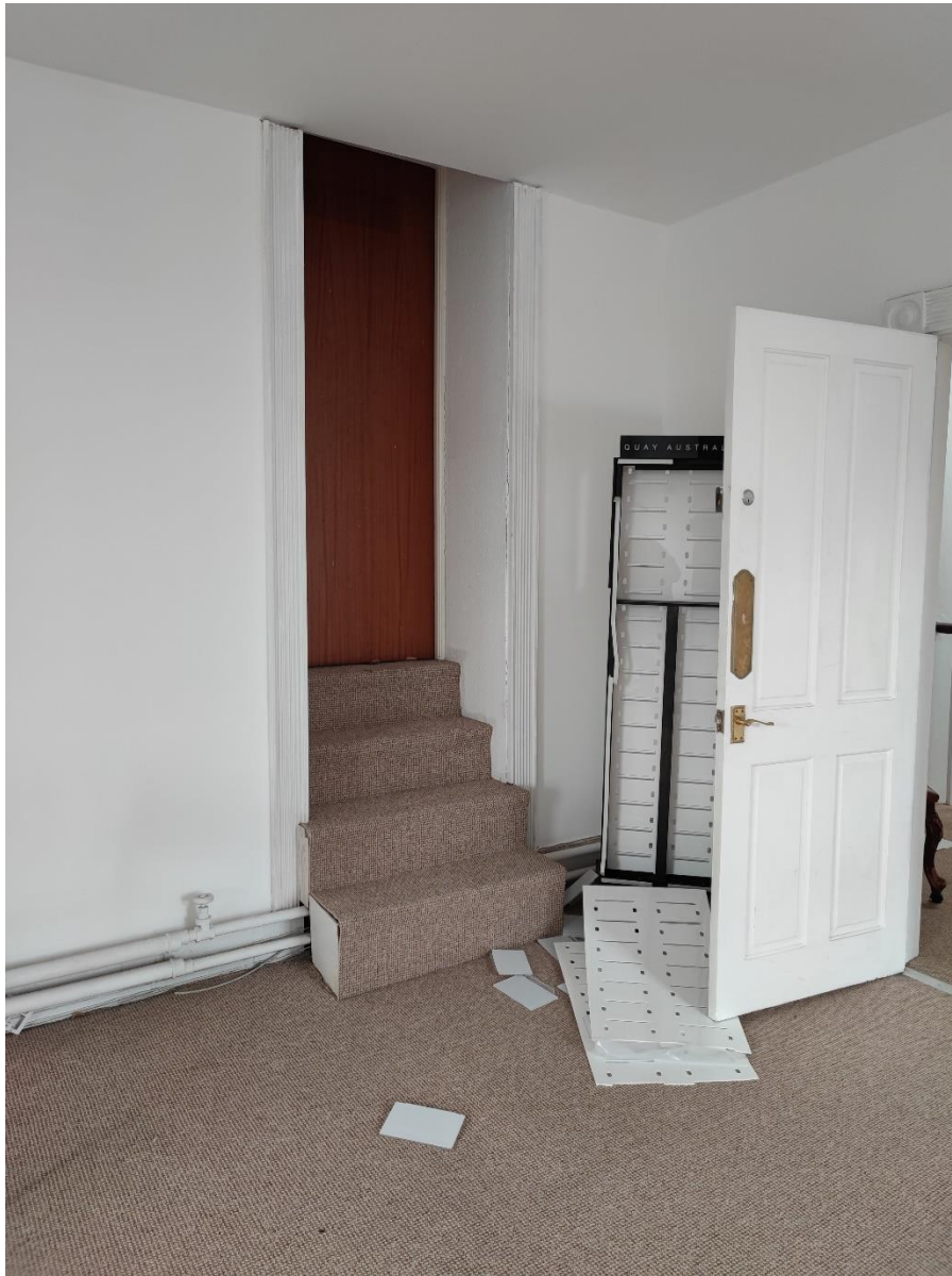
Figure 24 – View North from the front towards the existing passway to No 27 Ardwick Green North. Passway would be blocked, existing stair and door to be covered.
