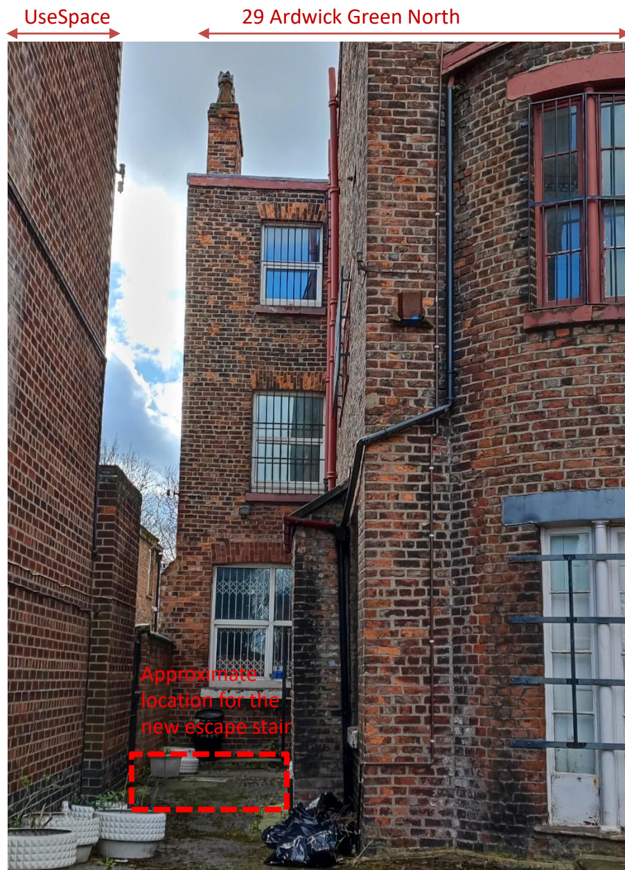
Figure 07 – View Southwest towards rear elevation Existing ground to be excavated for new escape stair to the basement association with handrail on the ground level
