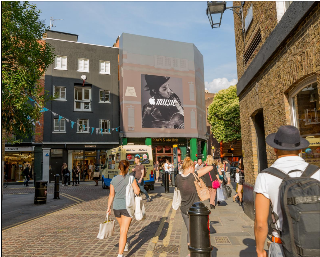
Fig. 3: Example of the aesthetic benefit potentially afforded by a scaffold shroud, Covent Garden
