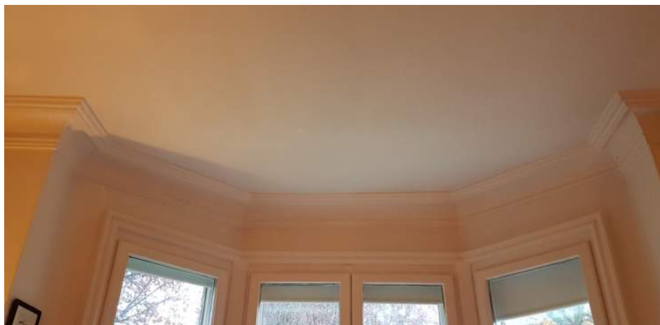
Figure 4: Internal view on opening through W gable wall into bay window showing patent lack of distress.
