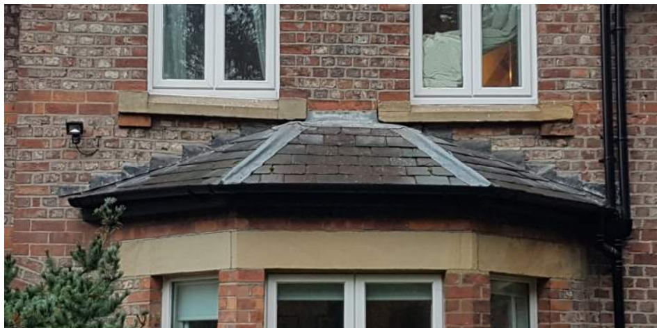
Figure 3: External view on significantly cranked geometry of the masonry skeleton (central pier translated downwards)
