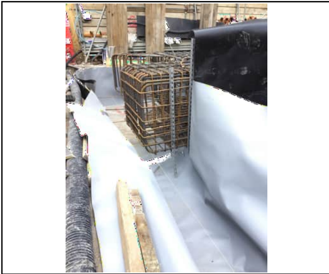
Visqueen Geoseal beneath ring beam
