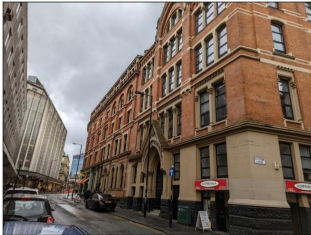
Image 4: View east up King Street West.
