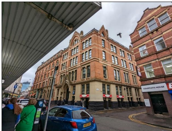
Image 2: Kings House - north and west elevations
