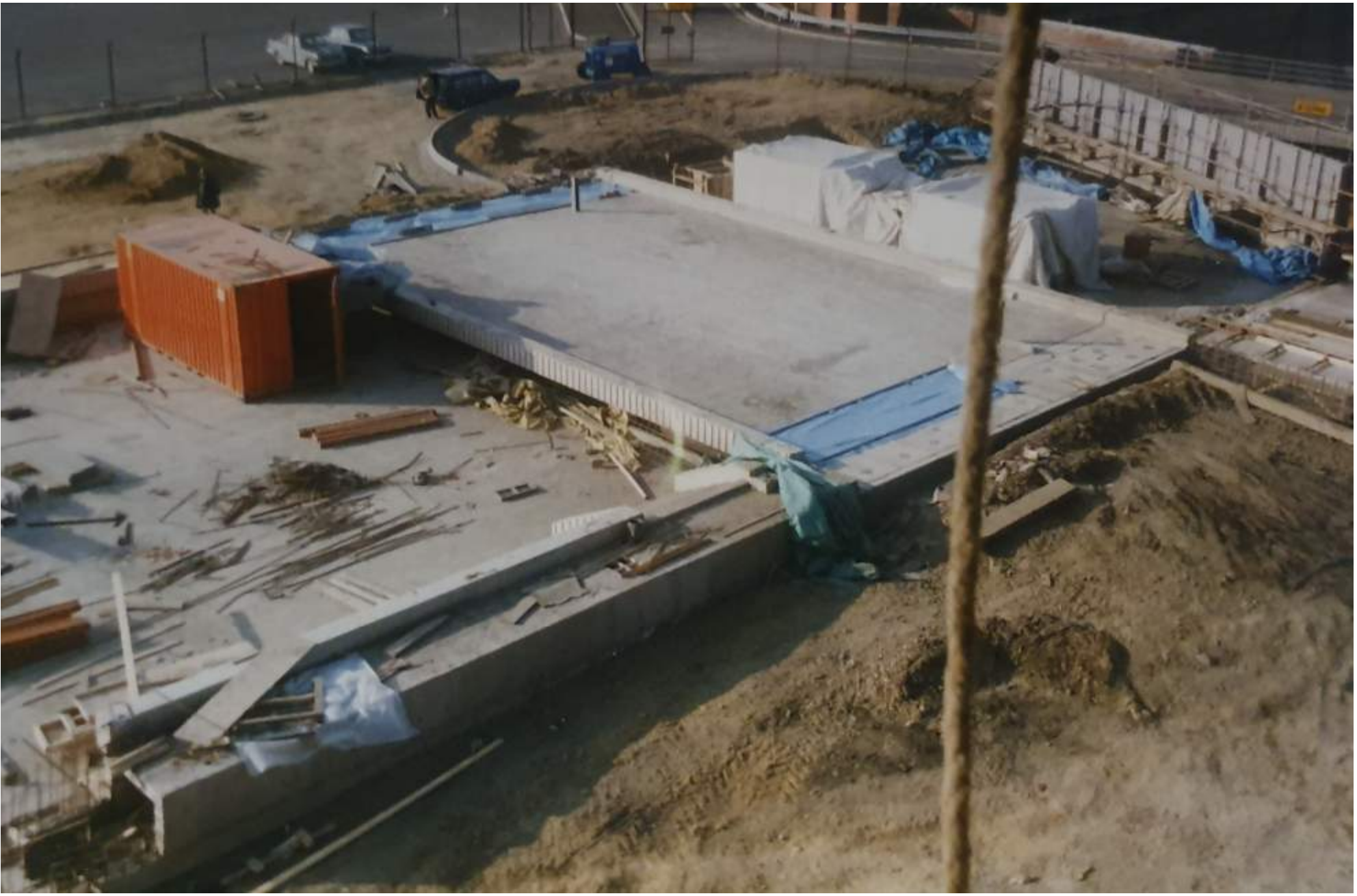
PHOTOGRAPH SHOWING COMPLETED BRIDGE 1, CONCRETE SLAB TO CAST-IRON ARCHES AND RC VENT DUCTS CIRCA 1985
