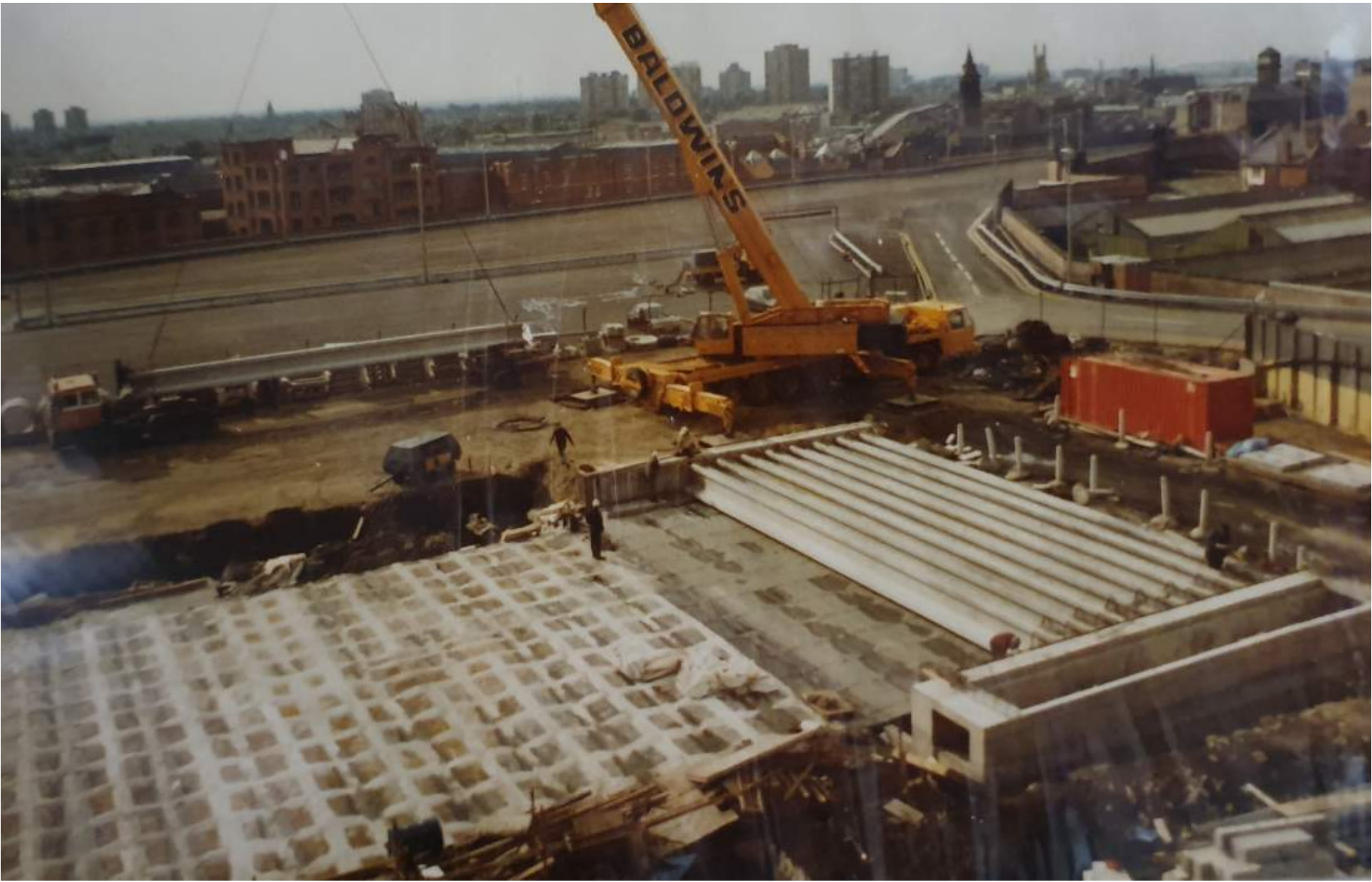
PHOTOGRAPH SHOWING BRIDGE 1 PRECAST CONCRETE INSTALLATION AND WATERPROOFING OF BUCKLE PLATES OVER CAST-IRON ARCHES CIRCA 1985
