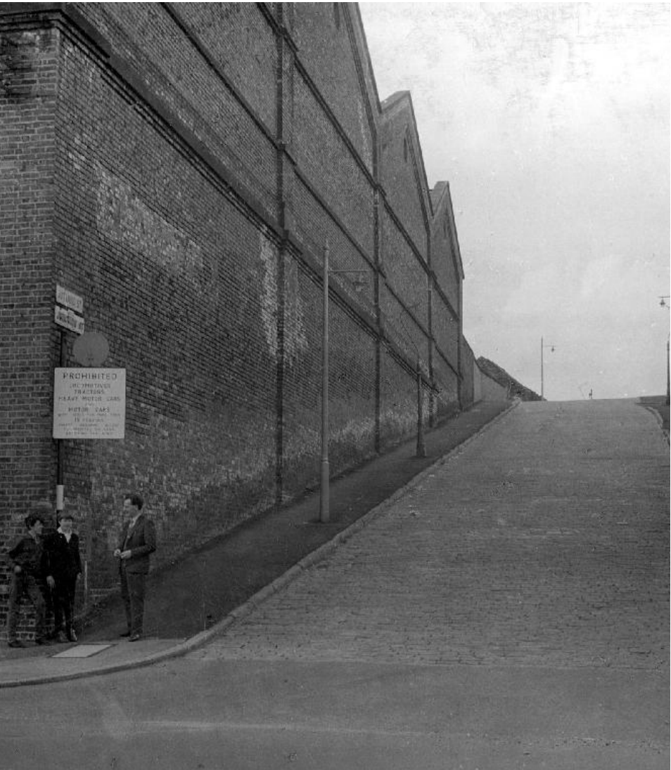
Corner of Jutland and Store Street
