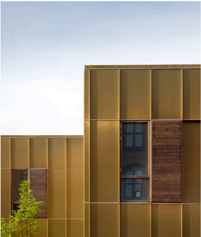
Flat panels with a standing seam joint
