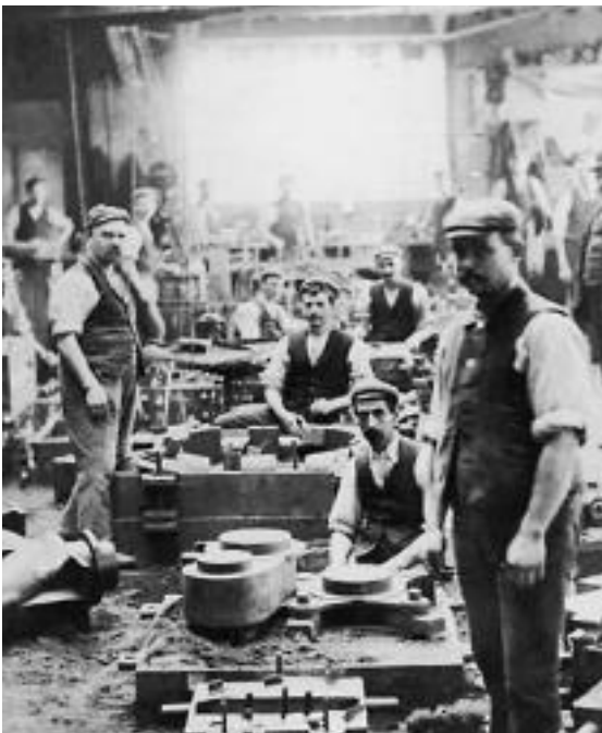
A typical Victorian foundry
