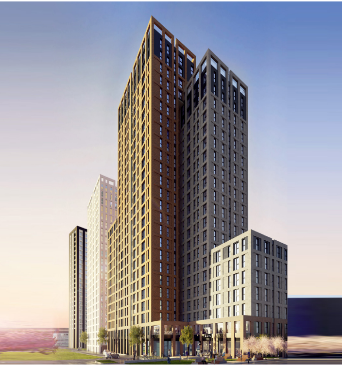
The Castings, Heyrod Street • Groundworks commenced May 2021 • 25 Storeys • 350 apartments
