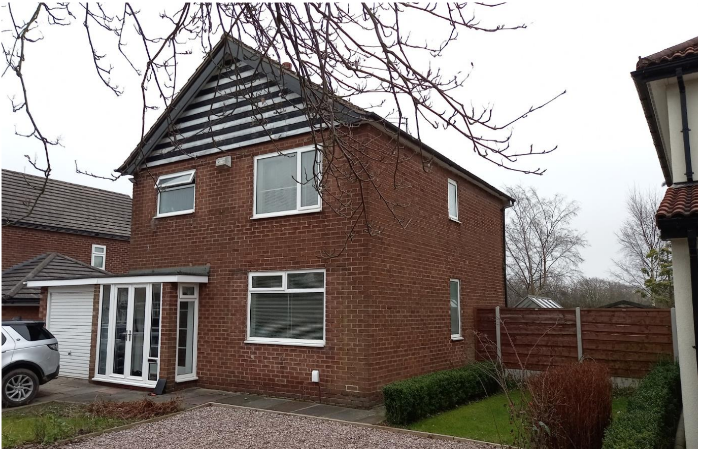
FRONT ELEVATIONS OF 41, PASTURE FIELD ROAD, PEEL HALL.
