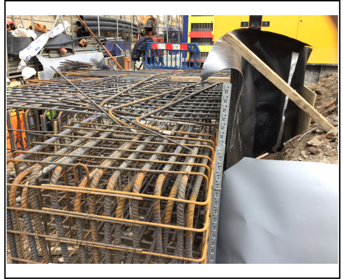
Visqueen Geoseal beneath
