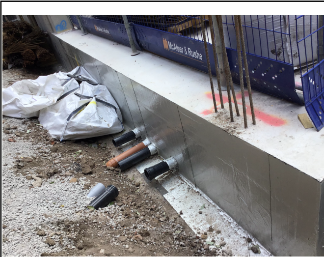
Perimeter detail sealed with no
