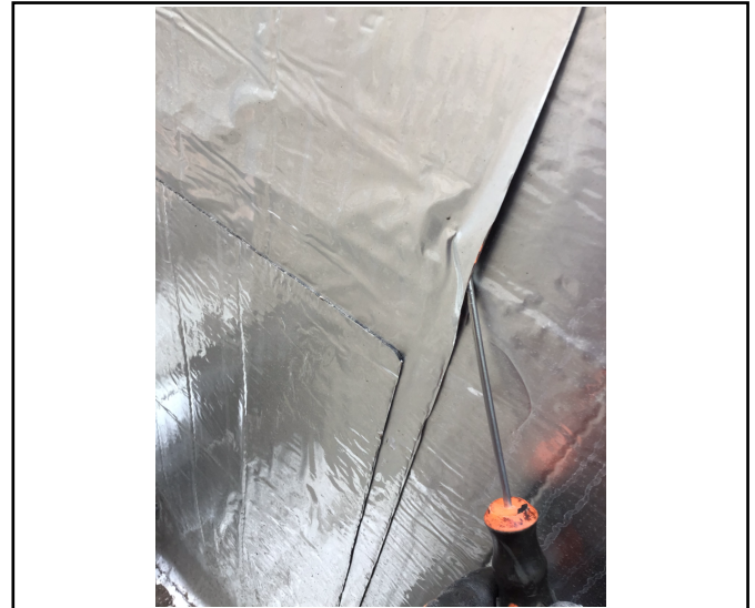
Pick and probe test to perimeter
