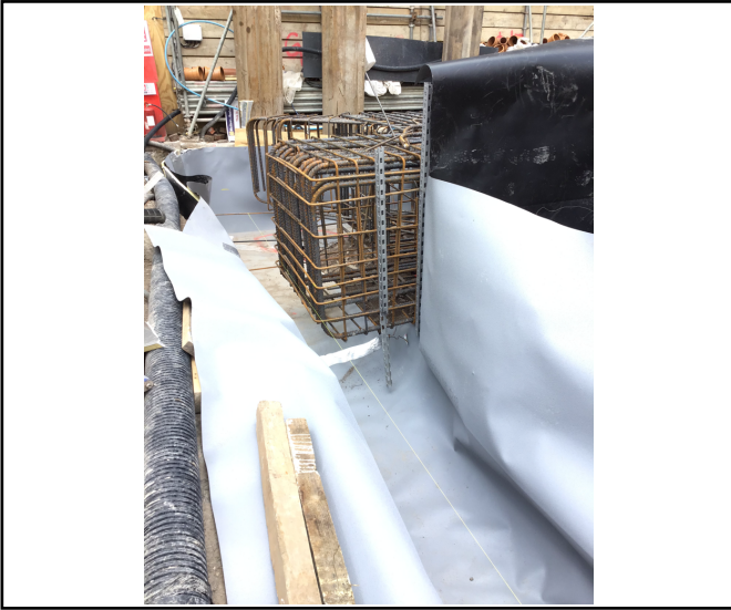
Visqueen Geoseal beneath ring beam
