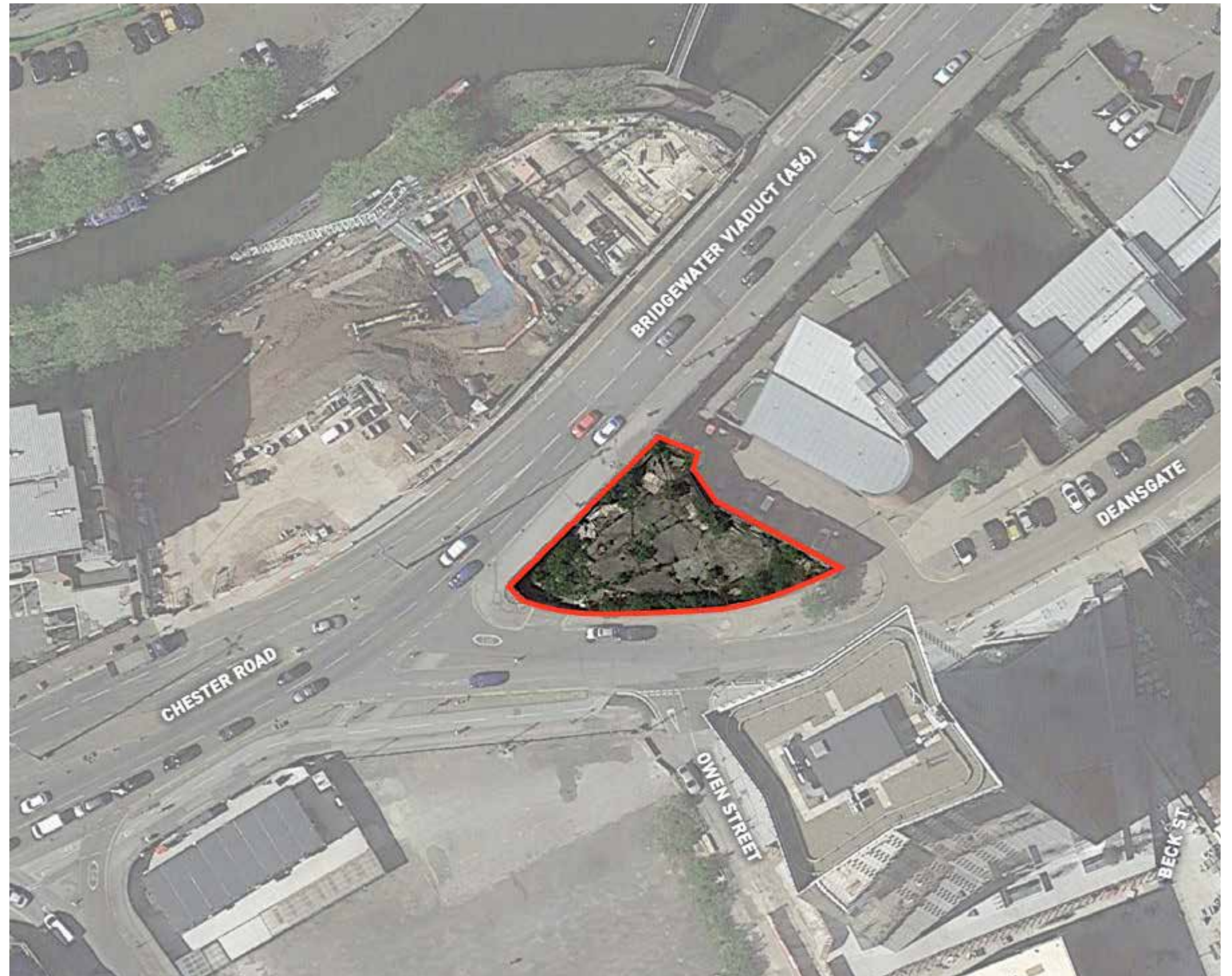
Aerial View of existing site.
