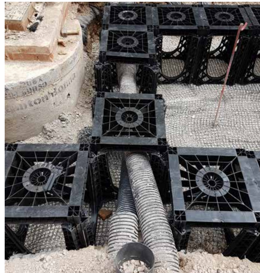
RootSpace Utility Integration at Kings Crescent, Hackney.
