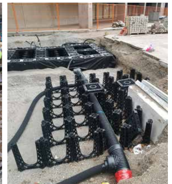
Jack Layton Ferry Terminal - Toronto, ON
