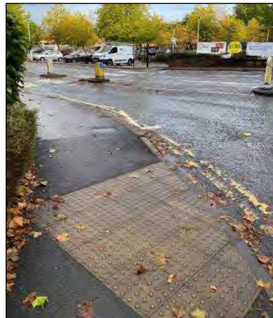
Figure 2.3 (left) – Dropped Kerb and Tactile Paving at Tesco / Parrs Wood Lane Junction (View from East)
