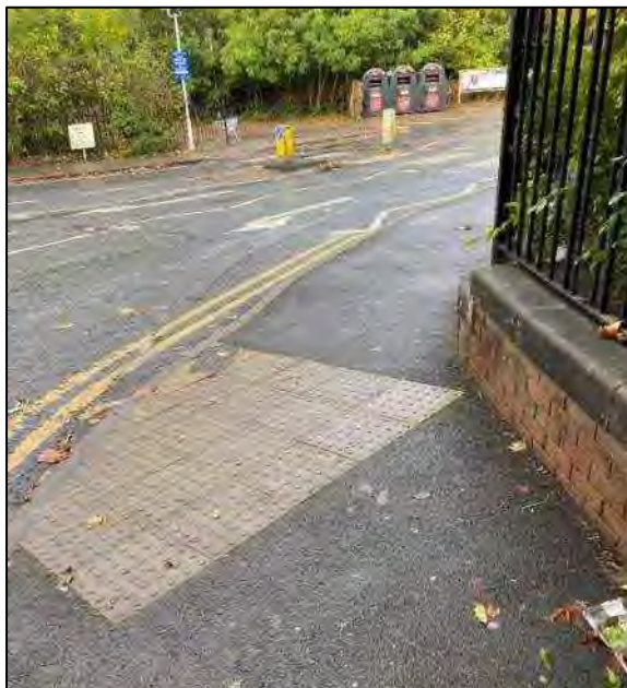
Figure 2.3 (left) – Dropped Kerb and Tactile Paving at Tesco / Parrs Wood Lane Junction (View from East)
