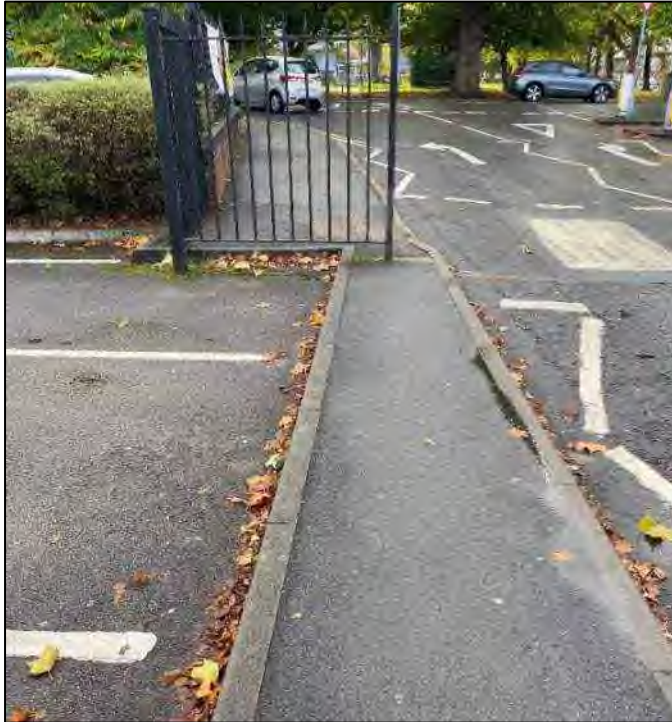
Figure 2.5 – Narrowing of Footway on Approach to Tesco (View from Within Tesco Looking out onto Parrs Wood Lane)
