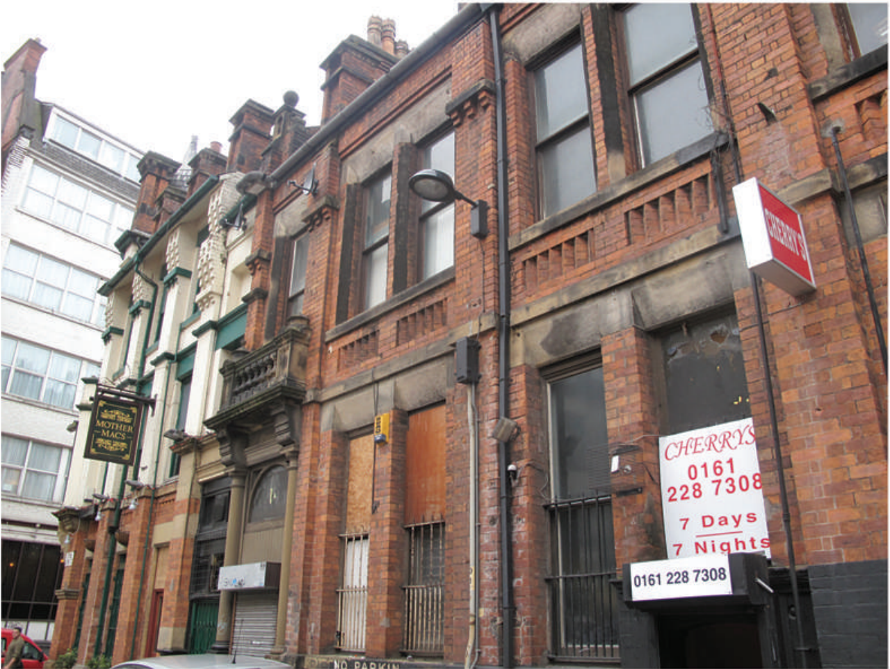
6. View of Mother's Macs Public House from Little Lever Street.
