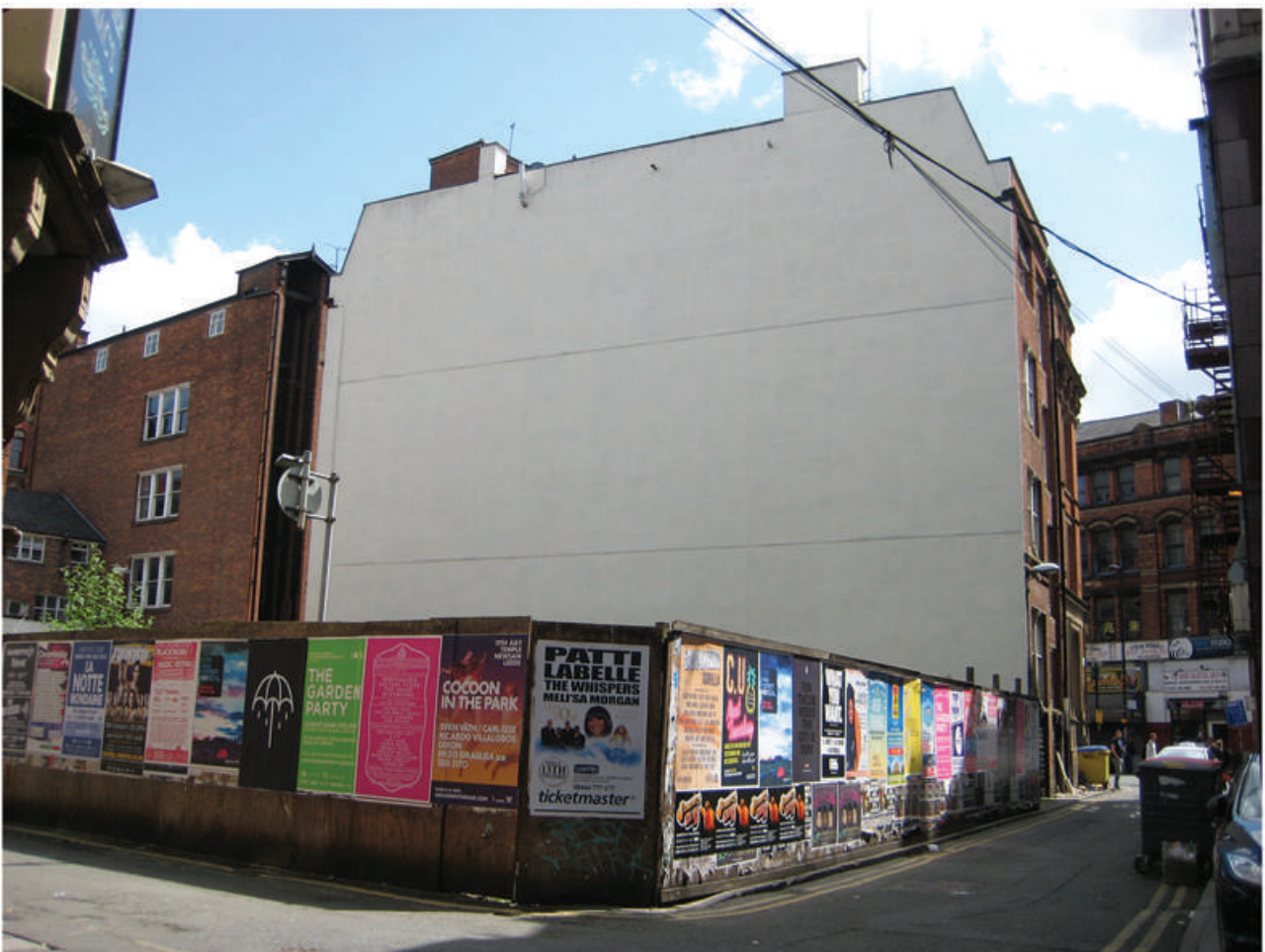
8. View of vacant site and Kingsley House (Grade II Listed).
