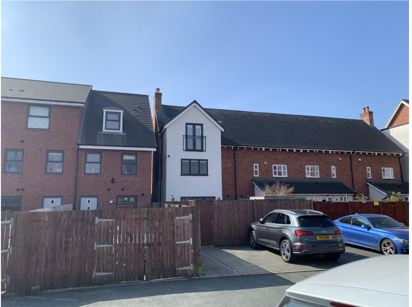
Photograph 2 Extension at 123 Nell Lane source: case officers photographs
