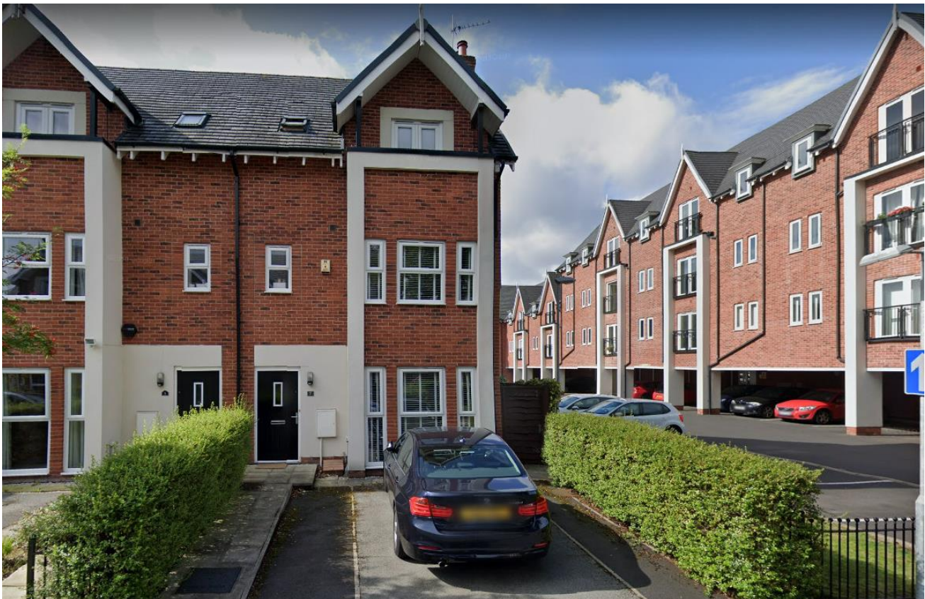
Photograph 1 Front elevation as viewed from High Trees Drive, Source: www.google.com/maps accessed 11.05.2022
