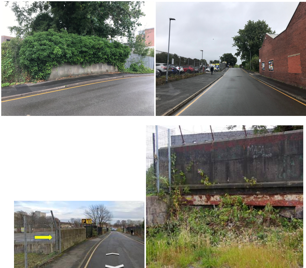
Figures 7,8 & 9,10 the southern parapet and the approach to the bridge from the west and the view looking south along the canal spur showing the 'barrier' now caused by the bridge
