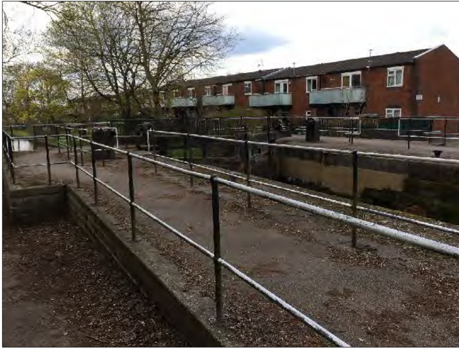
Figure 3.3: Pedestrian Bridges over the Rochdale Canal
