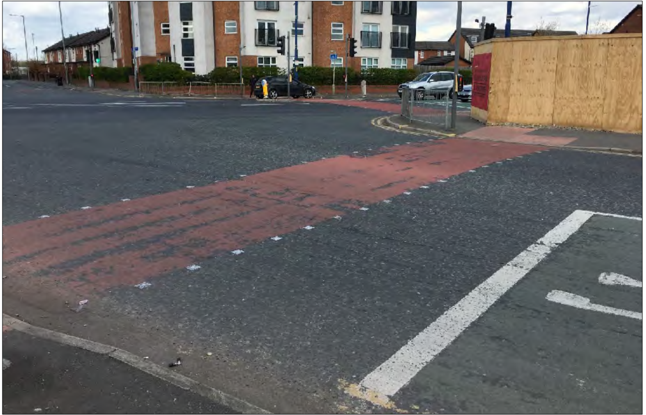
Figure 3.4: Pedestrian Infrastructure at the Dean Lane / A62 Oldham Road / Old Church Lane Junction
