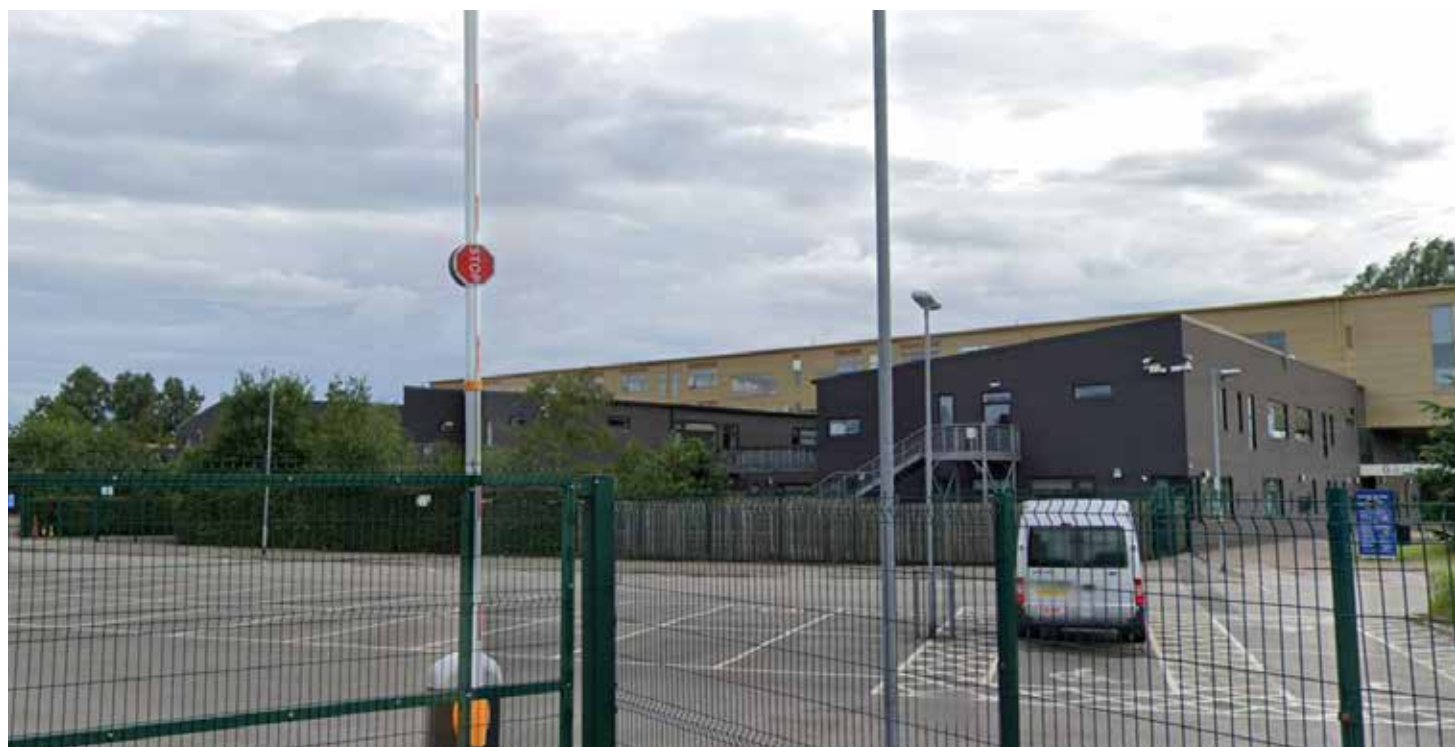
School Main Entrance
