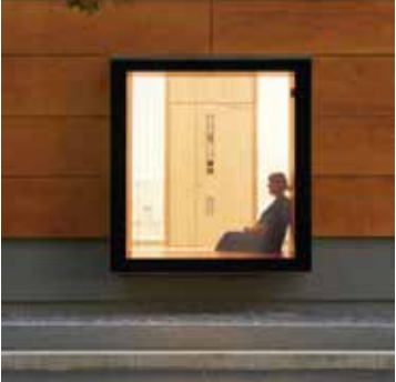
Projecting aluminium window surround
