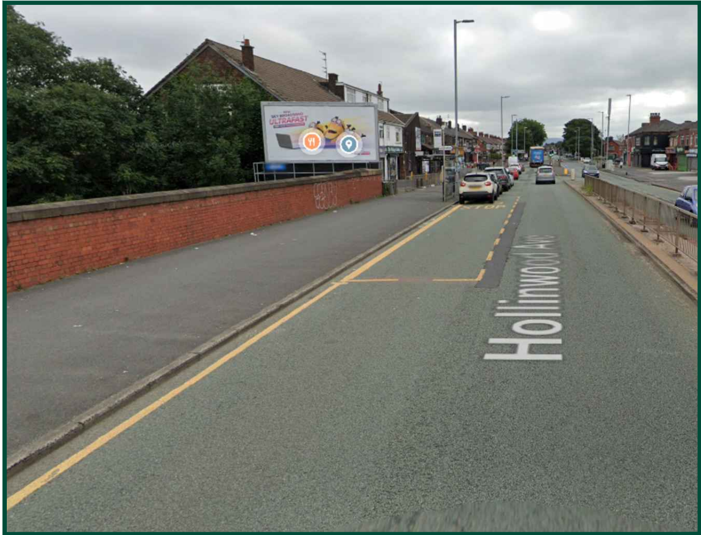
EXISTING SITE VIEW
