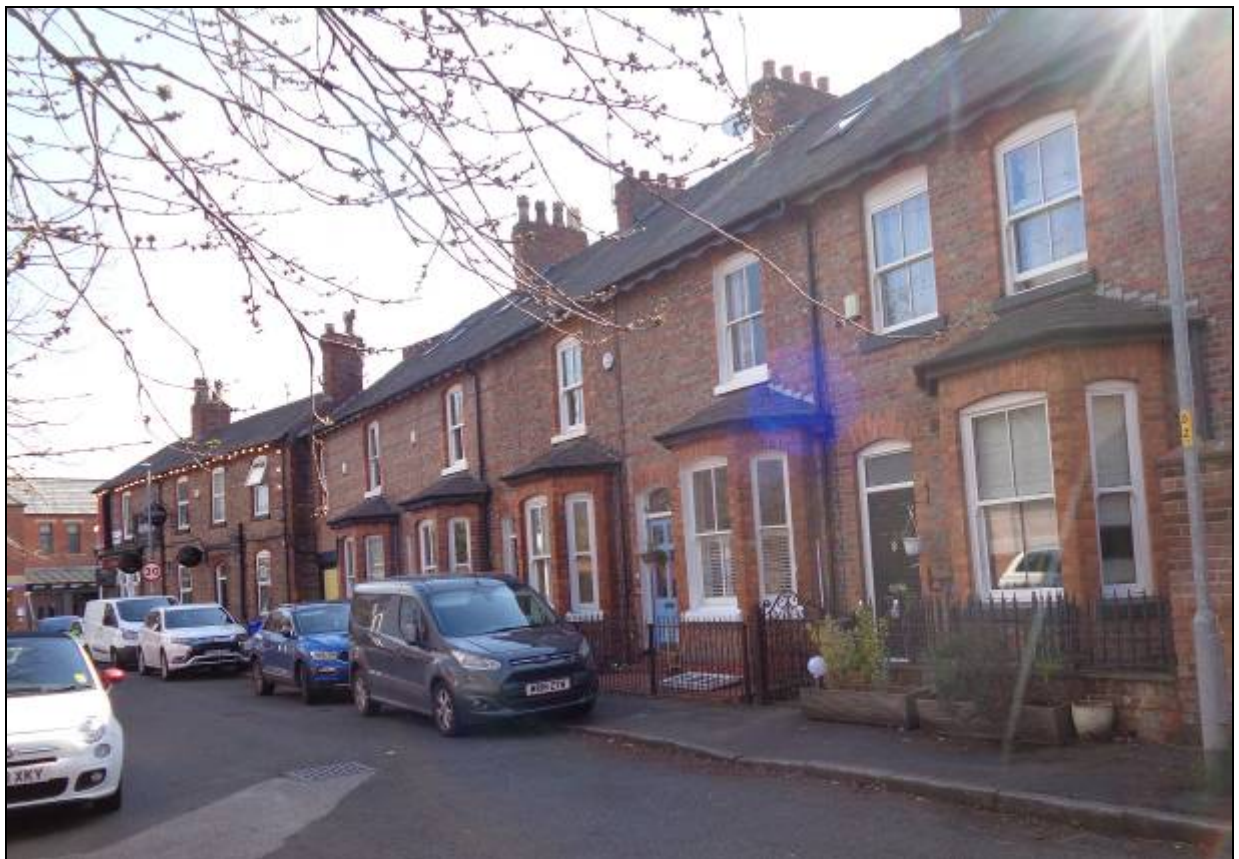
2. The property forms part of a late 19 th century terrace
