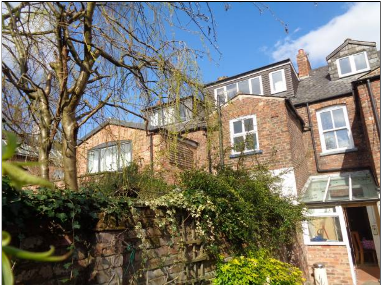
10. Existing full-width dormers at neighbouring properties
