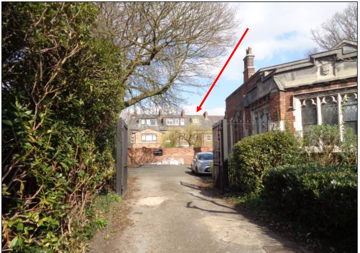
8. Distant view of the rear of the terrace from between Emmanuel Church and the Library
