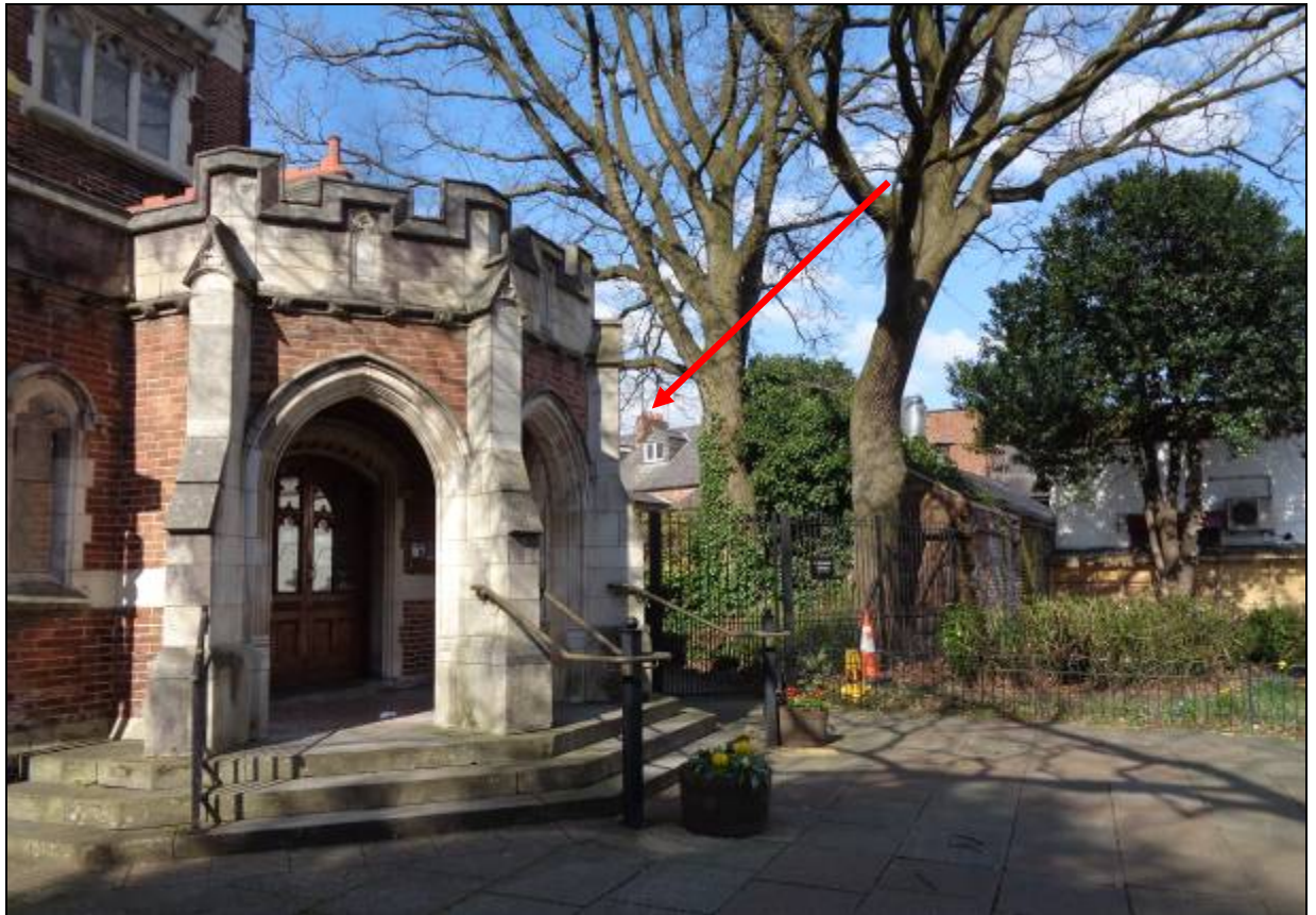
7. Glimpse of the roof from adjoining the Library
