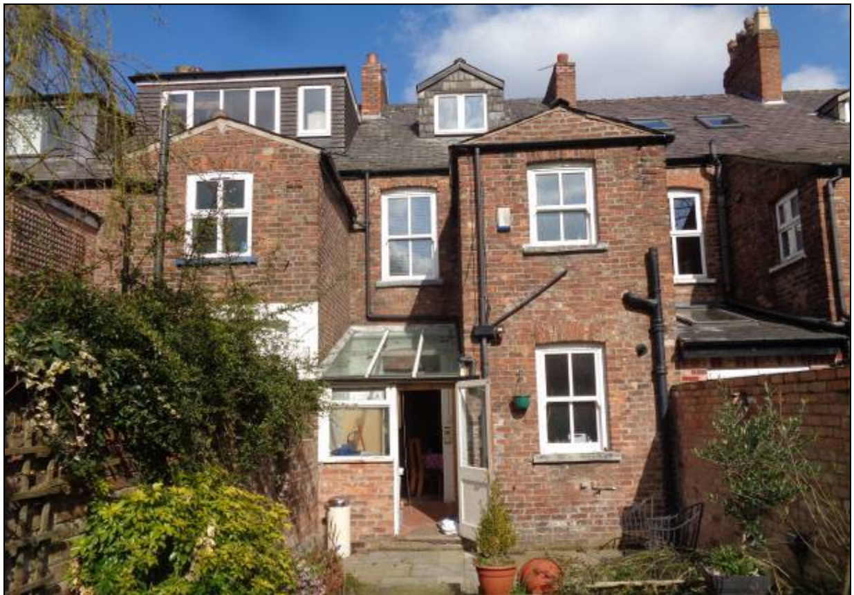
6. Rear of the application property, showing existing small dormer
