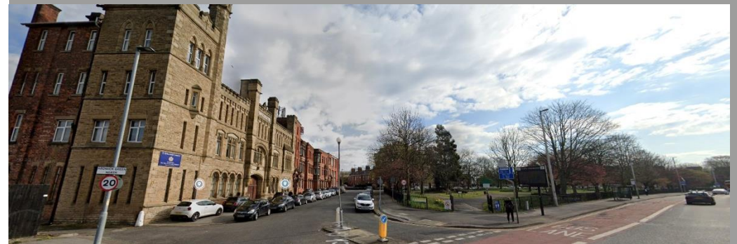
Figure 05 - View 1 | East from A6 to surroundings context
