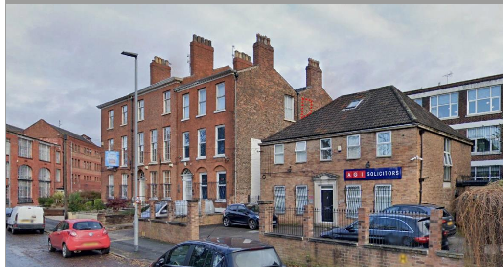
Figure 13 - View on Ardwick Green North towards 29 side elevation
