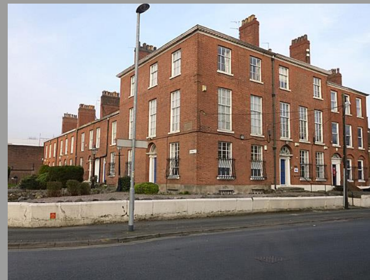
Figure 02 - Photo of corner of Manor Street and Ardwick Green North
