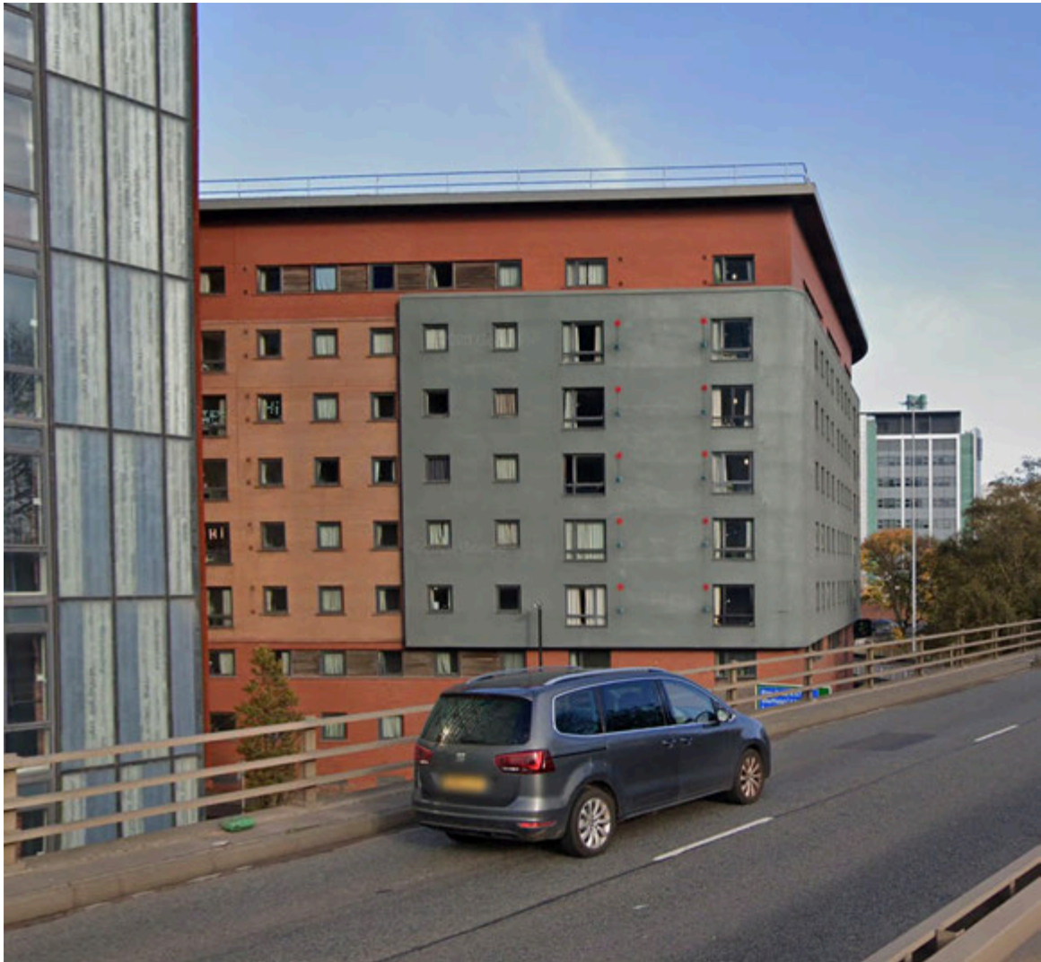
EXISTING (View from A635(M))
