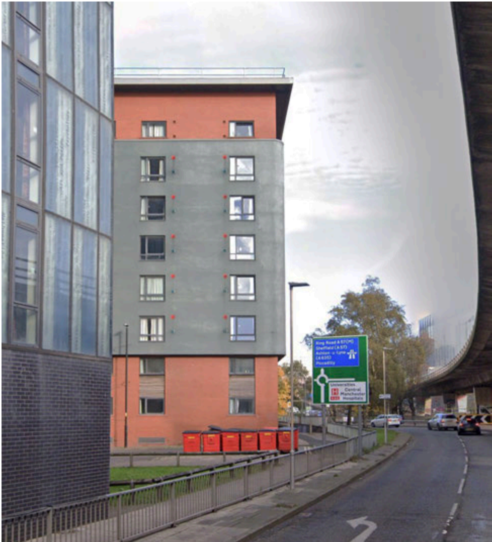
EXISTING (View from A5103)
