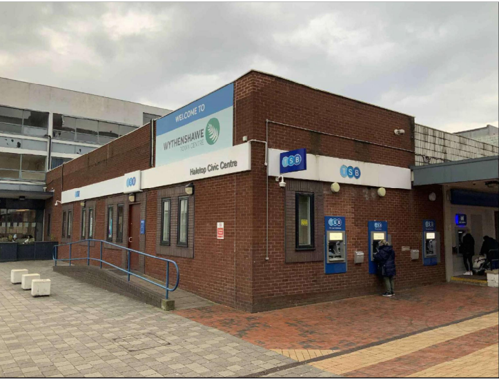
STREET SCENE TO TSB BRANCH
