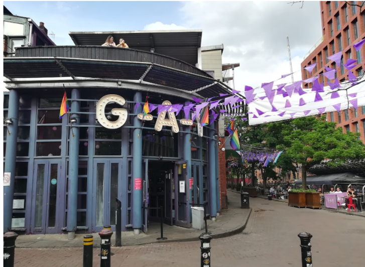
Figure 2: Rooftop/Terrace bar – G-A-Y Manchester
