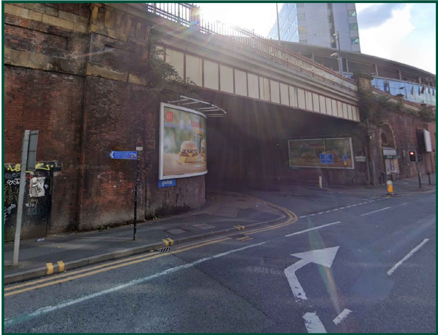
EXISTING SITE VIEW
