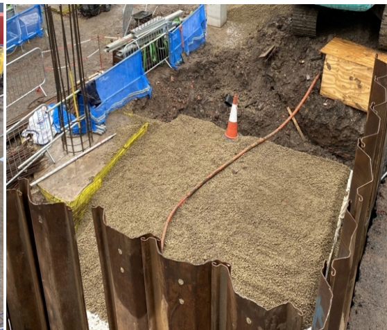
Figure 3 - Backfill
