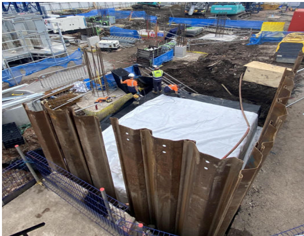
Figure 2 - Completion and Backfill
