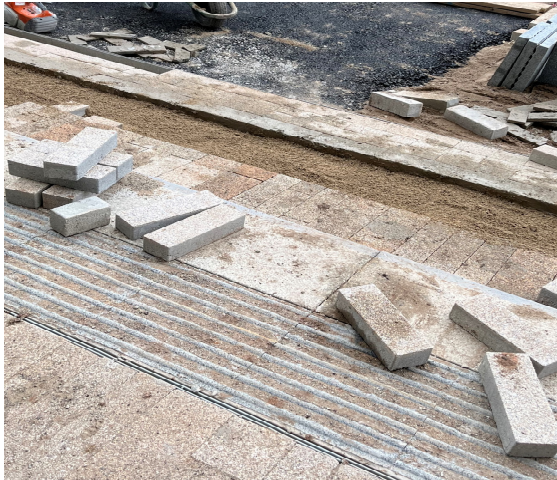
Figure 4 - Slot Drain Installation at Top Step
