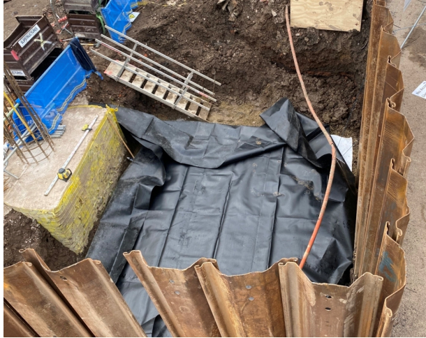
Figure 1 - Attenuation Tank Formation
