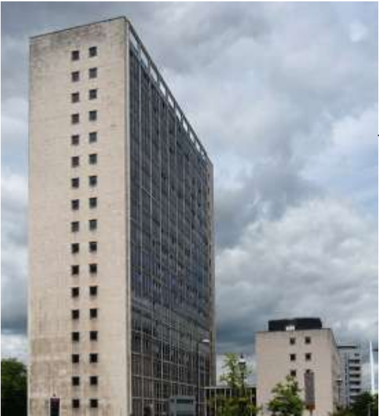
ALBERT BRIDGE HOUSE 1 Bridge Street
