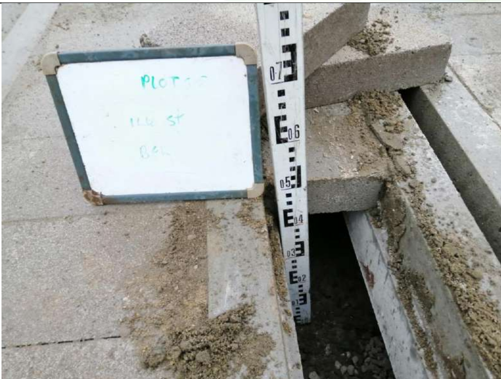
Photograph 4: Validation of Sub-Floor Void Space (min 150 mm)
