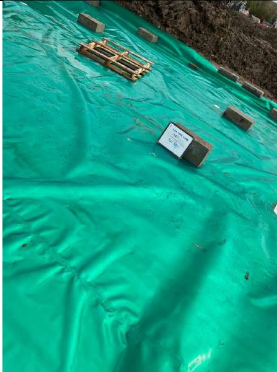
Photograph 5: Validation of Gas Membrane Installation
