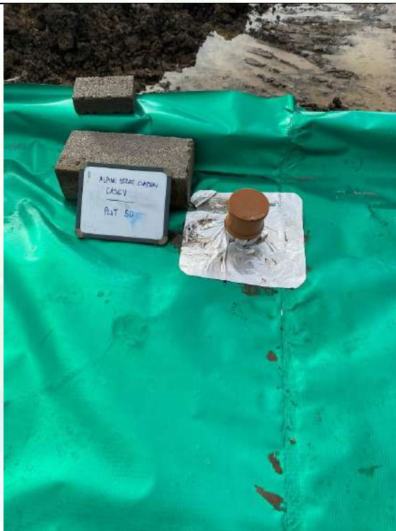
Photograph 6: Validation of Gas Membrane Installation
