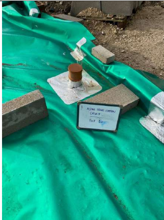
Photograph 7: Validation of Gas Membrane Installation
