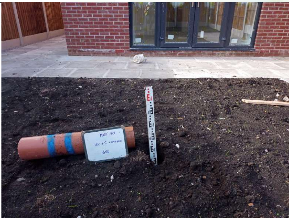
Photograph 2: Validation of Garden Capping Thickness
