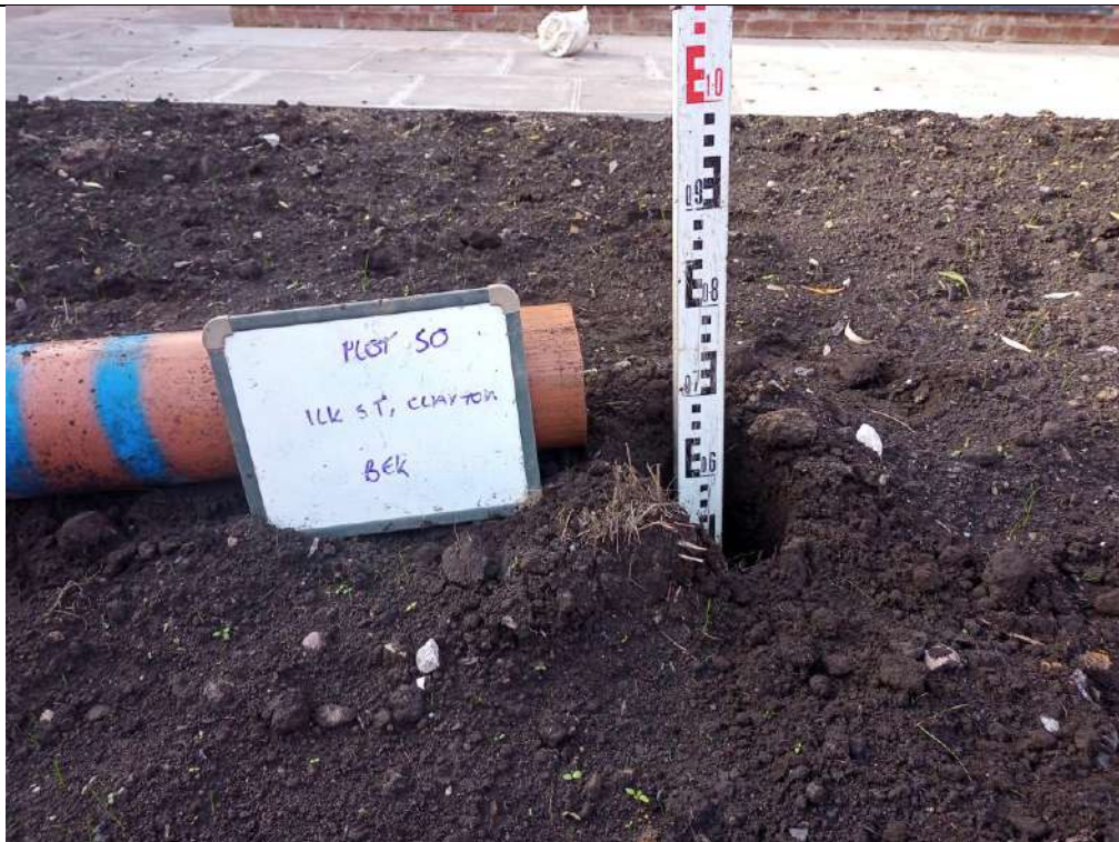
Photograph 1: Validation of Garden Capping Thickness
