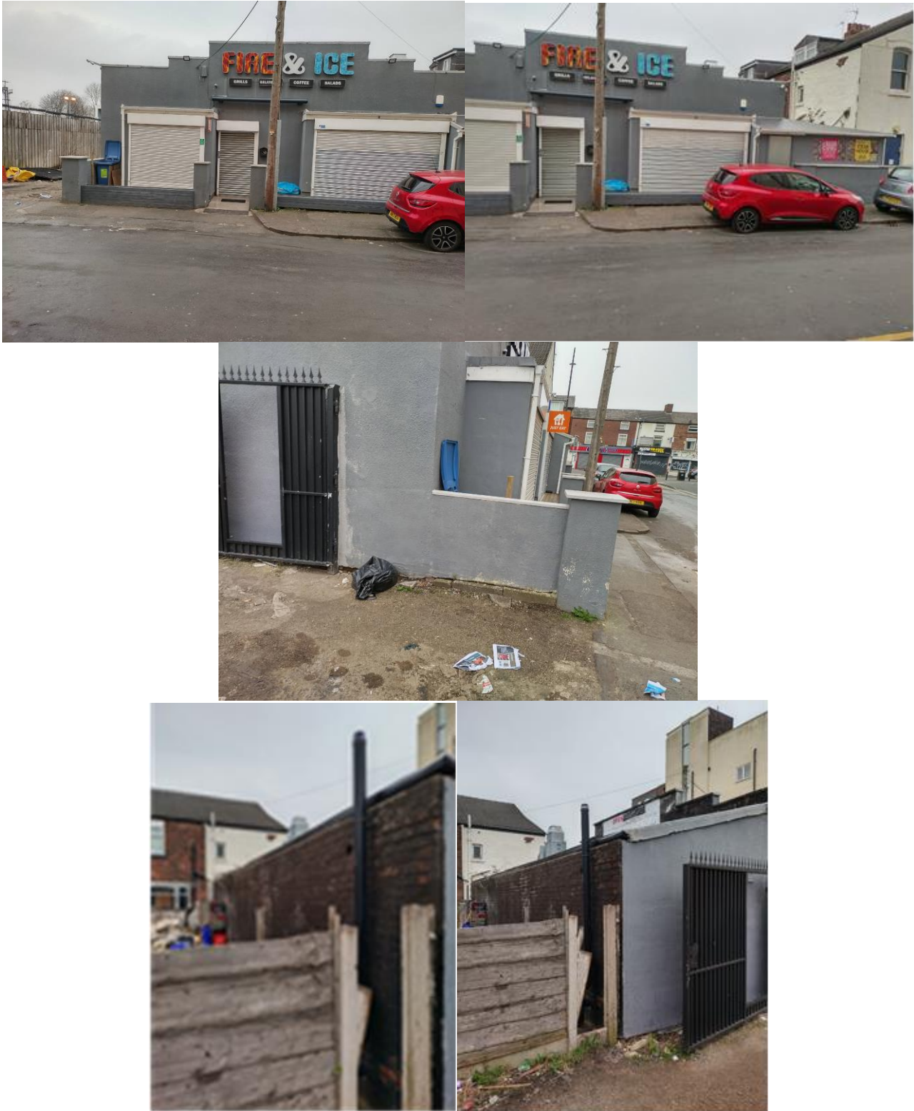
Fig. 1 – Views of the application site
