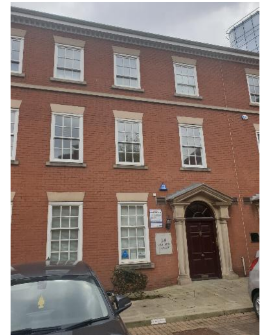
Entrance from Oxford View
