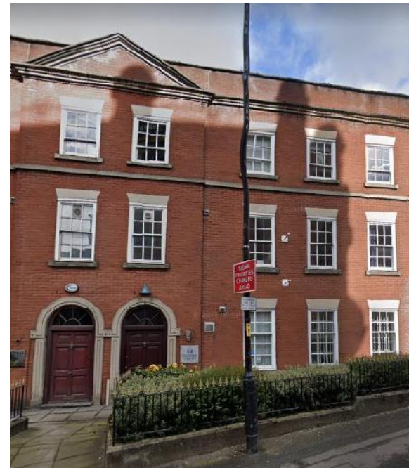
Entrance from Chepstow Street
