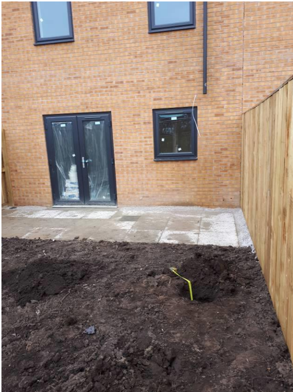
Photograph 11: Plot 274 Validation Pit Location 2
