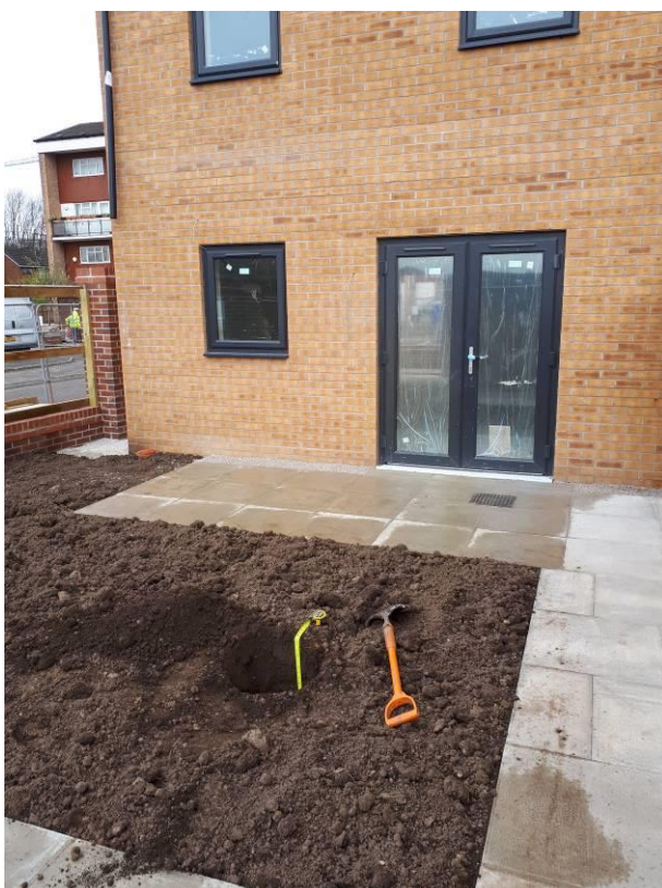
Photograph 15: Plot 275 Validation Pit Location 2
