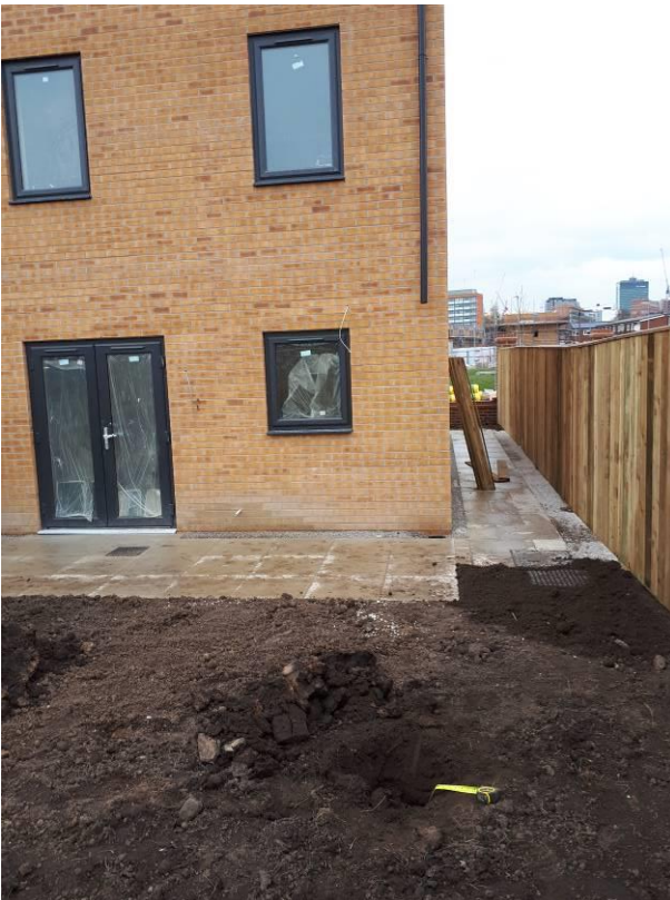
Photograph 7: Plot 273 Validation Pit Location 2
