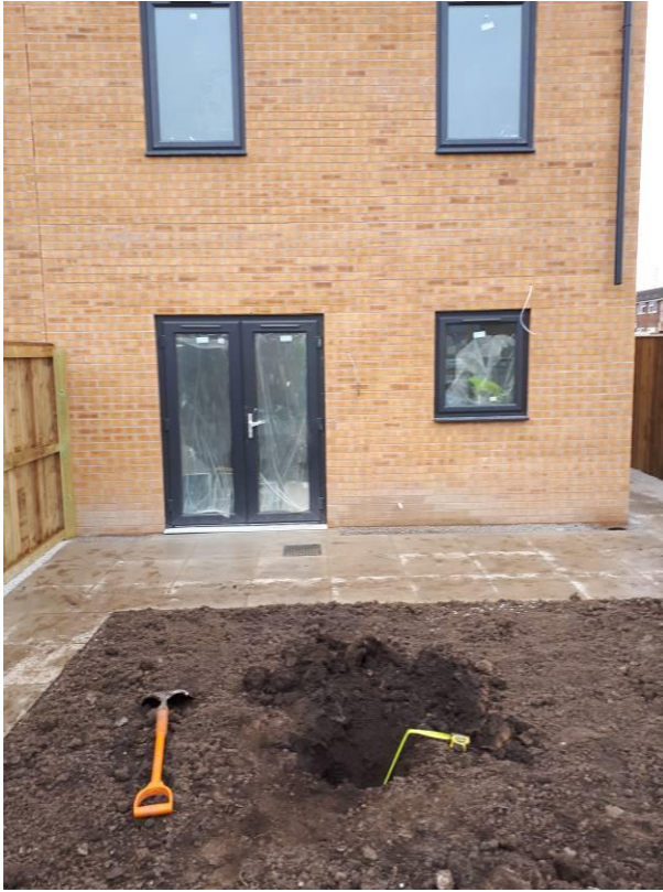
Photograph 5: Plot 273 Validation Pit Location 1
