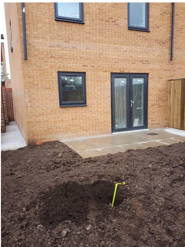
Photograph 13: Plot 275 Validation Pit Location 1
