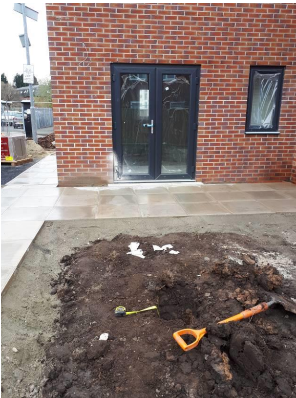
Photograph 3: Plot 220 Validation Pit Location 2
