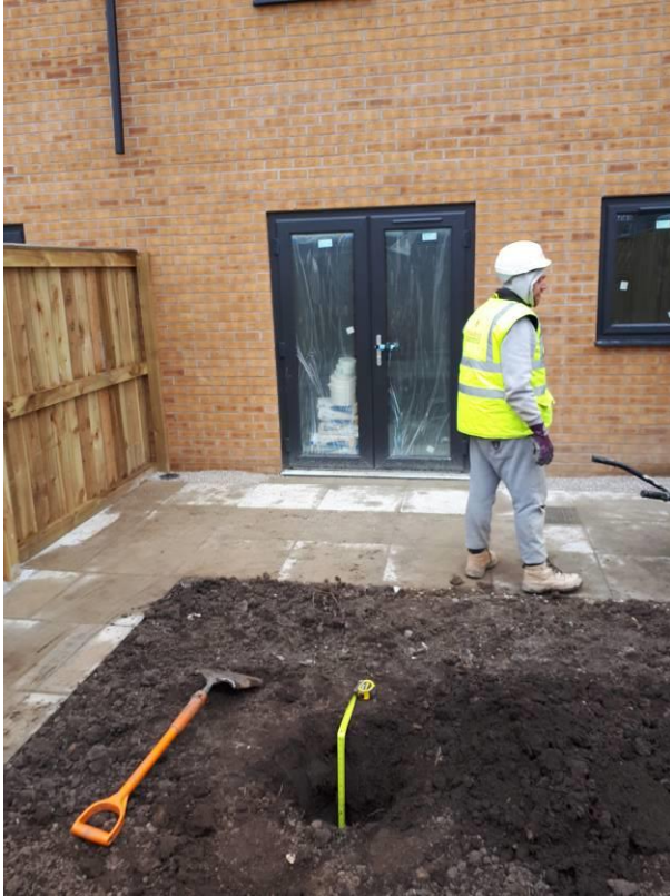
Photograph 9: Plot 274 Validation Pit Location 1
