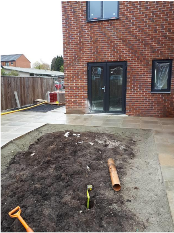
Photograph 1: Plot 220 Validation Pit Location 1
