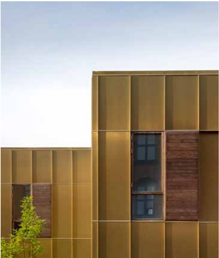
Flat panels with a standing seam joint
