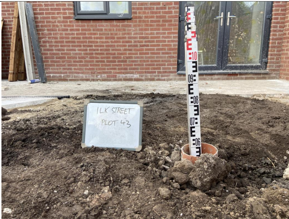
Photograph 1: Validation of Garden Capping Thickness
