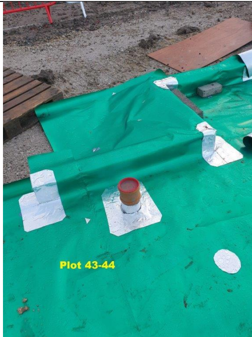
Photograph 5: Validation of Gas Membrane Installation (Please note, plots 43 and 44 are semidetached and were validated together. Gas membranes are satisfactory within both plots)
