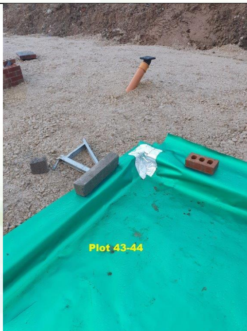
Photograph 6: Validation of Gas Membrane Installation (Please note, plots 43 and 44 are semidetached and were validated together. Gas membranes are satisfactory within both plots)
