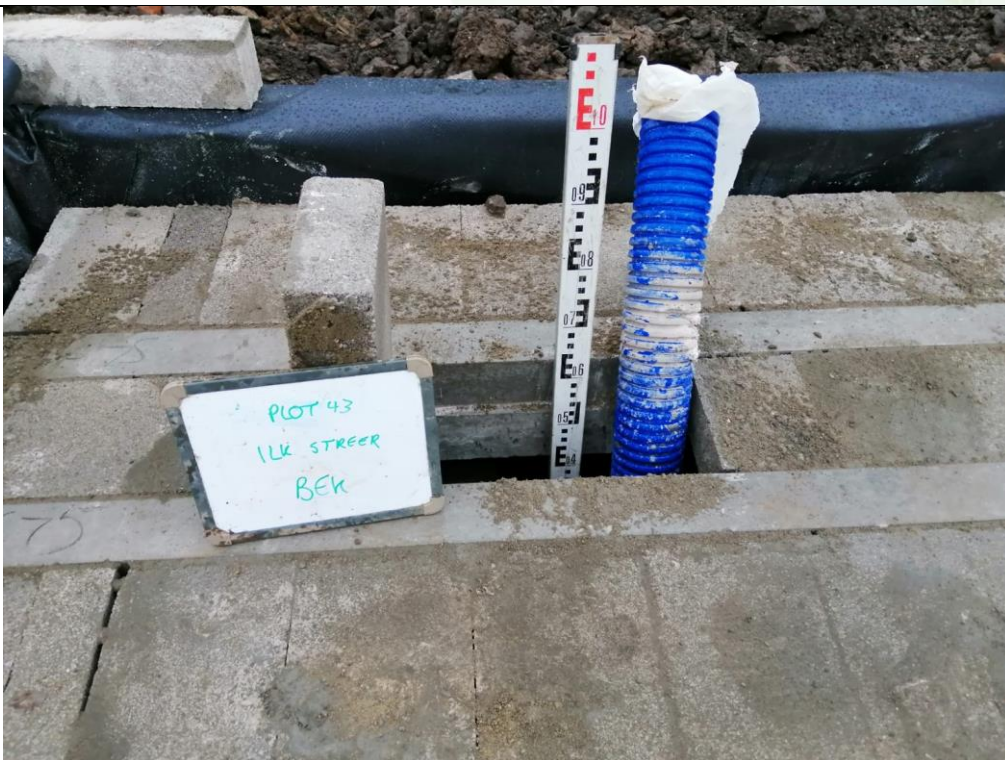
Photograph 4: Validation of Sub-Floor Void Space (min 150 mm)
