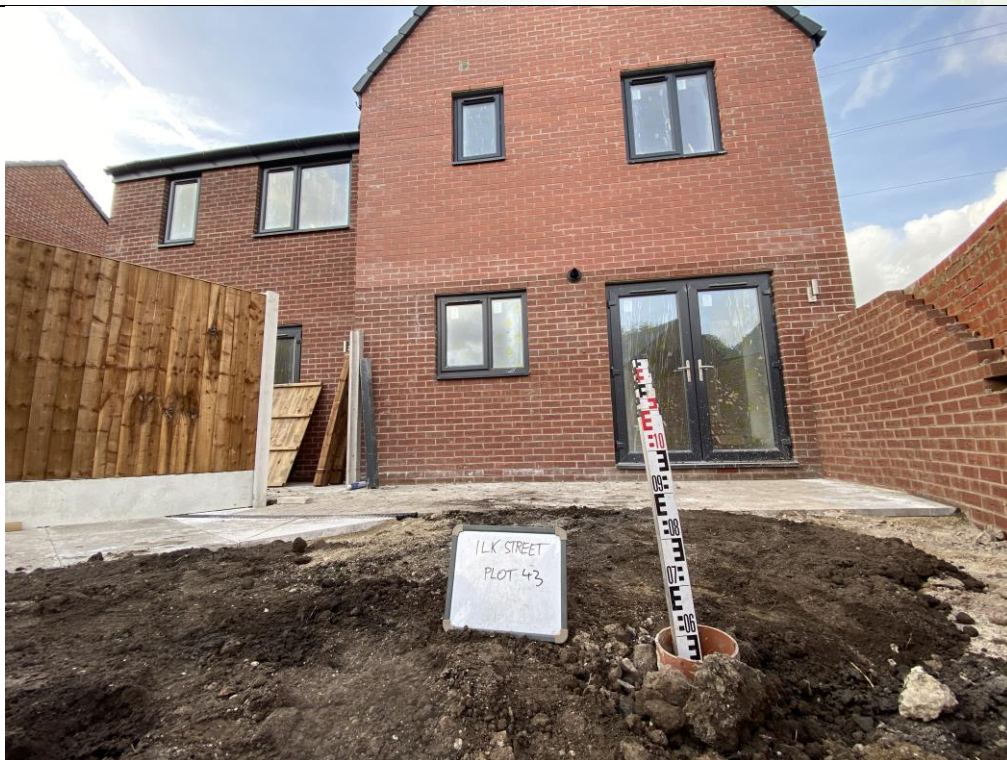
Photograph 2: Validation of Garden Capping Thickness
