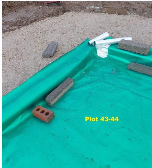
Photograph 7: Validation of Gas Membrane Installation (Please note, plots 43 and 44 are semidetached and were validated together. Gas membranes are satisfactory within both plots)
