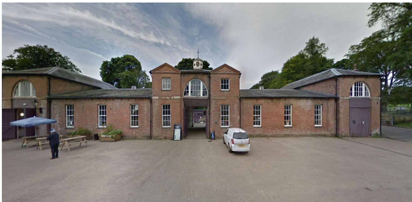
Figure 2: View of the Front Elevation of the Heaton Park Farm Centre (Former Stable Block).
