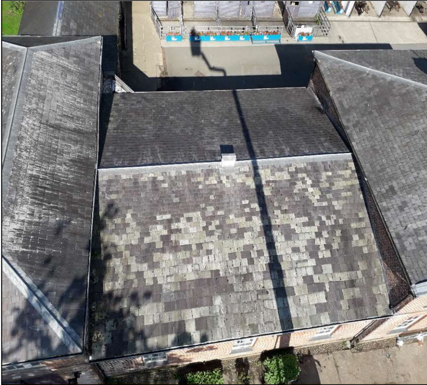
Figure 5: Aerial View of Roof Area 2 – Proposed Re-roofing
