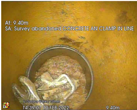
SW1 US RE6_9-40m_143907.jpg, 00:00:35, 9.40 m Survey abandoned, CONCRETE AN CLAMP IN LINE
