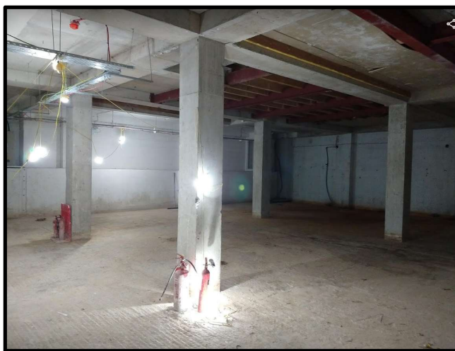
Image 1: Existing vacant basement
