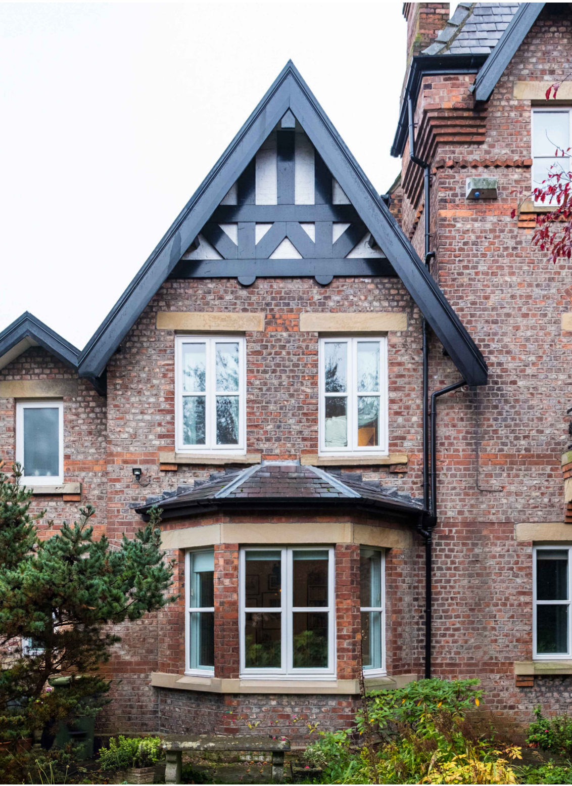
Existing West Elevation Photograph Not to Scale
