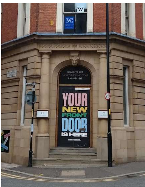
Image 5: Existing pedestrian access
