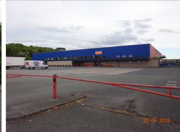
Pic 10 shows a view of the Booker Wholesale premises on the southern side of Lawton Road, opposite the proposed development site.
