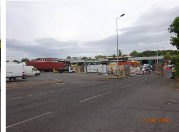
Pic 3 taken from just inside the existing southern market entrance shows the view looking east across the proposed development site towards the perimeter with Press Street.
