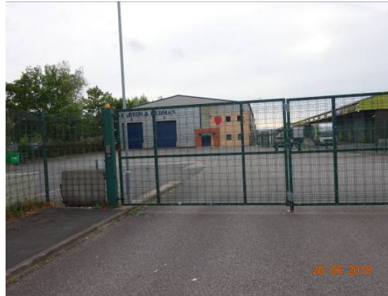
Pic 2 shows the existing secure eastern perimeter of the Barton and Redman site and the current entrance.
