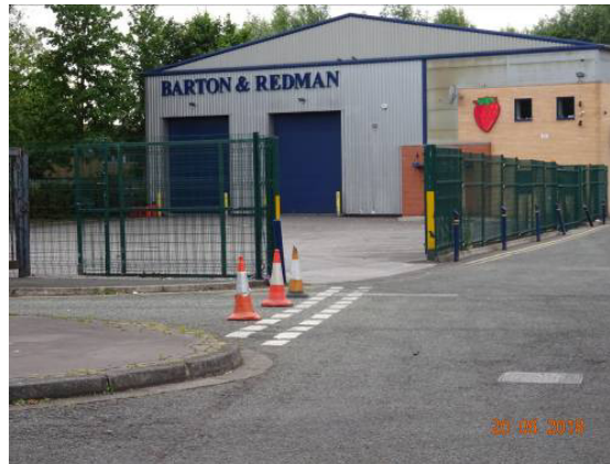
Pic 5 shows the existing northern perimeter of the Barton and Redman site looking west.
