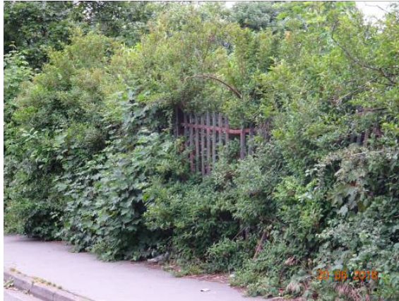
Pic 7 shows a close up view of the perimeter seen in the previous photograph, showing the existing metal palisade fencing within the shrubbery.
