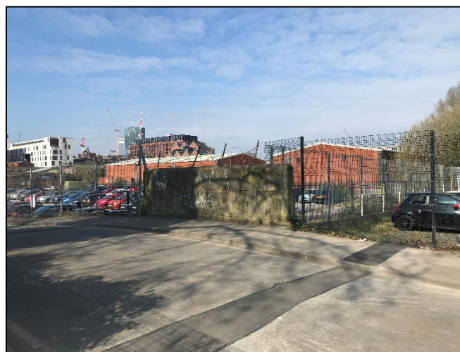
Figure 4: The Northern elevation of the bridge viewed from jersey Street.
