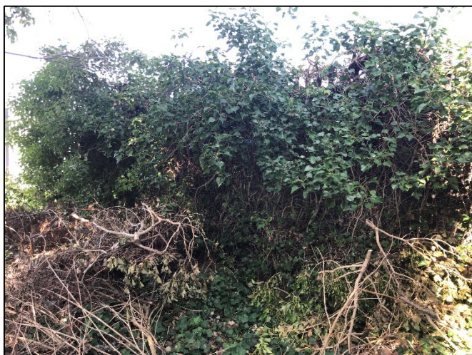
Figure 4: The southern side of the bridge was covered in ivy.
