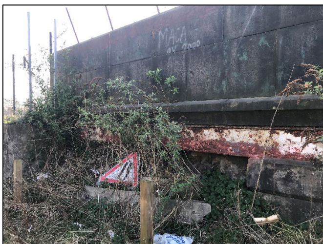
Figure 3: The photo shows the northern elevation of the bridge.
