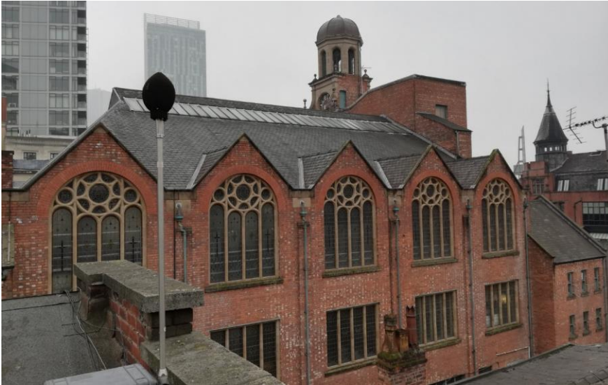
Figure B2 Photograph denoting unattended monitoring position L2
