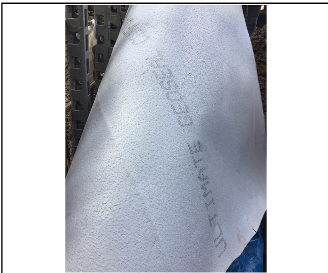
Visqueen Geoseal Ultimate used
