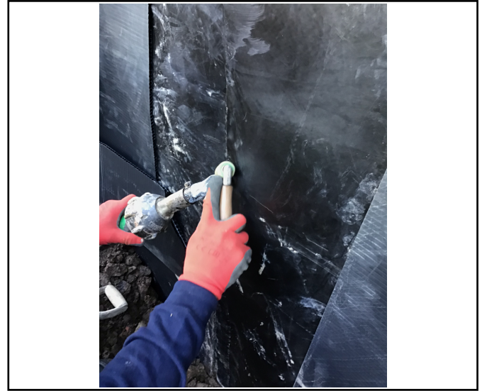
Hot weld in before extrusion
