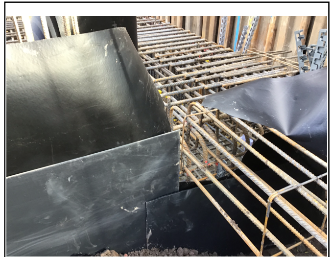
Membrane cut around ring beam
