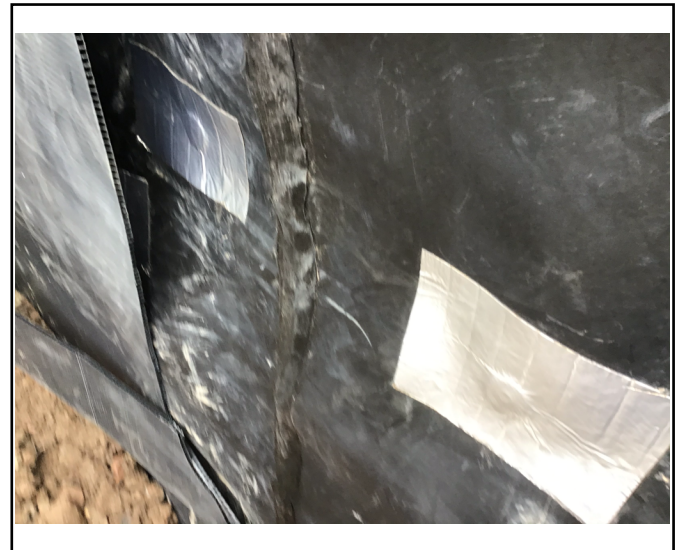
Pegs installed either side of
