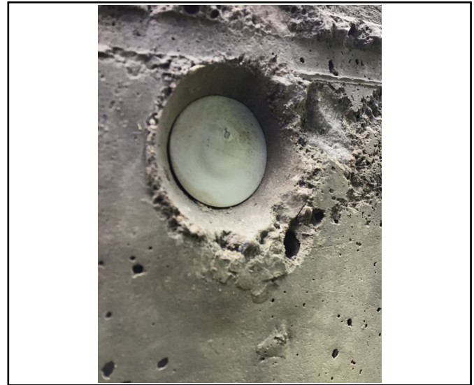
Dividag holes plugged with rubber
