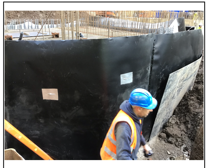
Pegs to bed in concrete sealed
