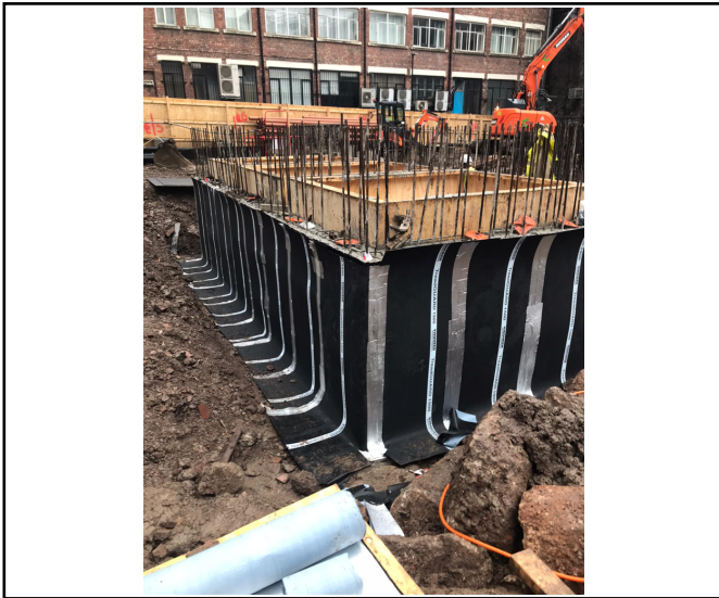
Core protected with protective boarding
