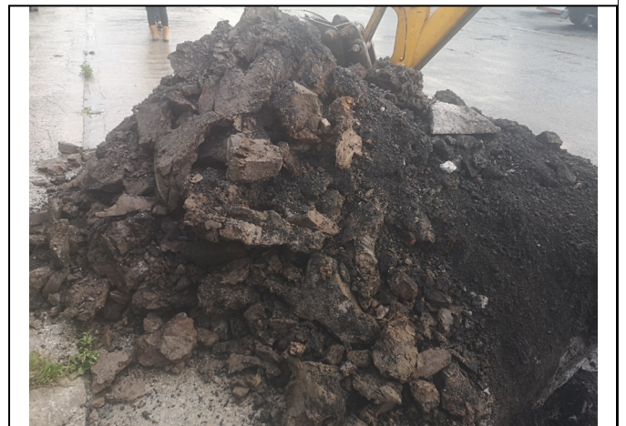
Trial Pit 207 Spoil
