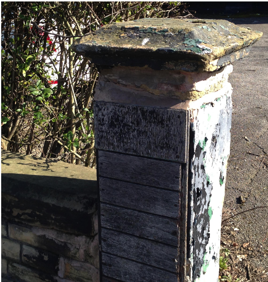
Photos showing the poor condition of the previous gatepost in 2014
