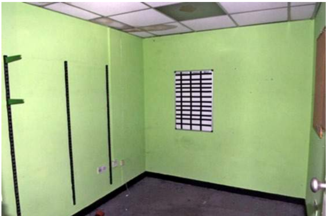
Plate 21. Structure B west end staff room at the west end of the Phase II section (facing south-east)
