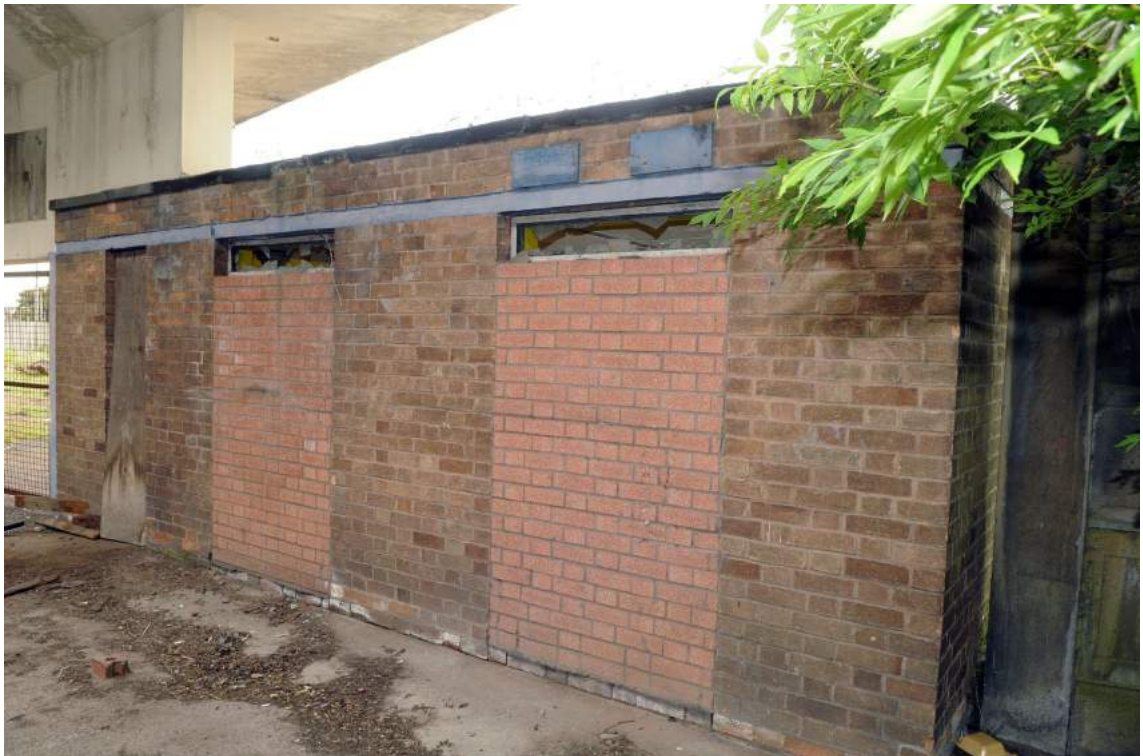
Plate 5: Structure A, north-east elevation of the west booth (facing south)
