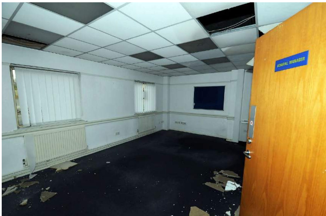
Plate 39. Structure B east end, General Manager's office (facing north-east)
