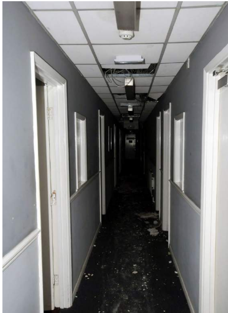
Plate 38. Structure B east end, Phase II offices to the right, Phase IV offices to the left (facing west)
