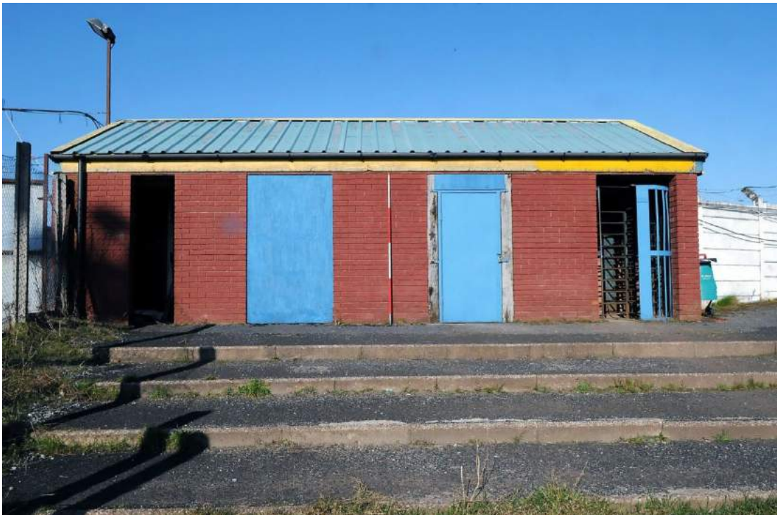
Plate 61. Structure C, south elevation (facing north)
