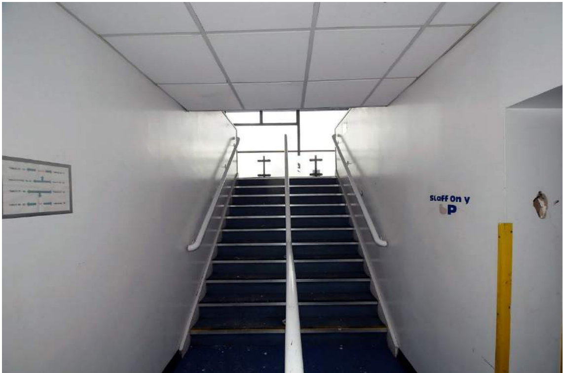
Plate 32. Structure B central, stair access to the track (facing south)
