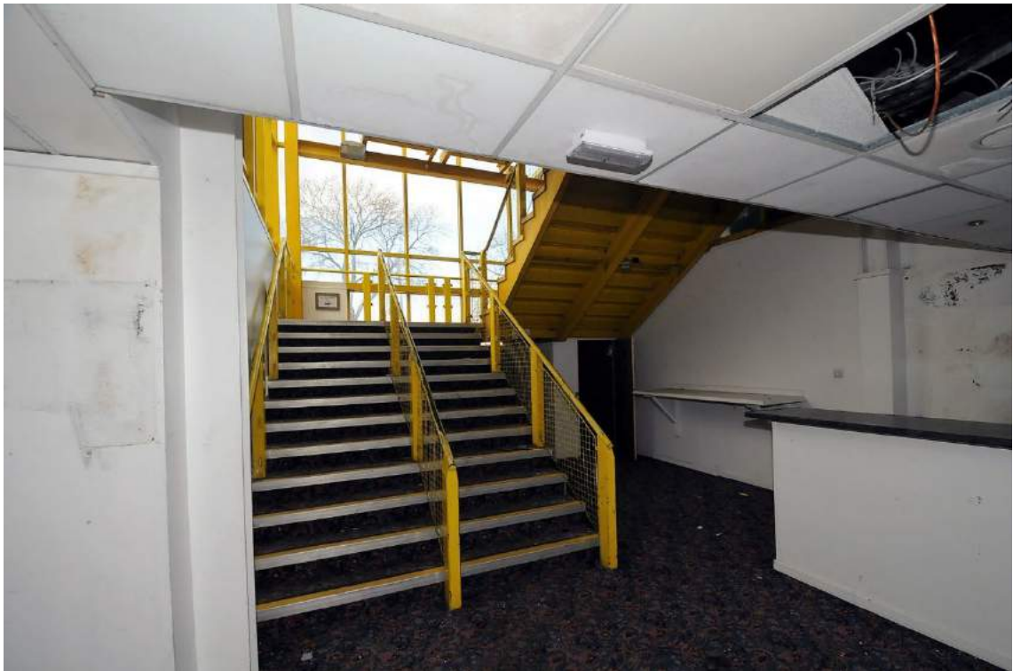
Plate 36. Structure B central, Phase IV staircase (facing north)
