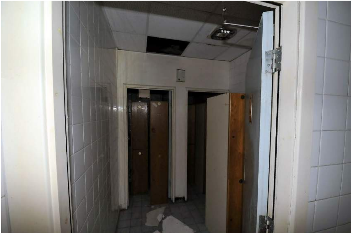
Plate 24. Structure B west end Phase IV WC facilities (facing west)
