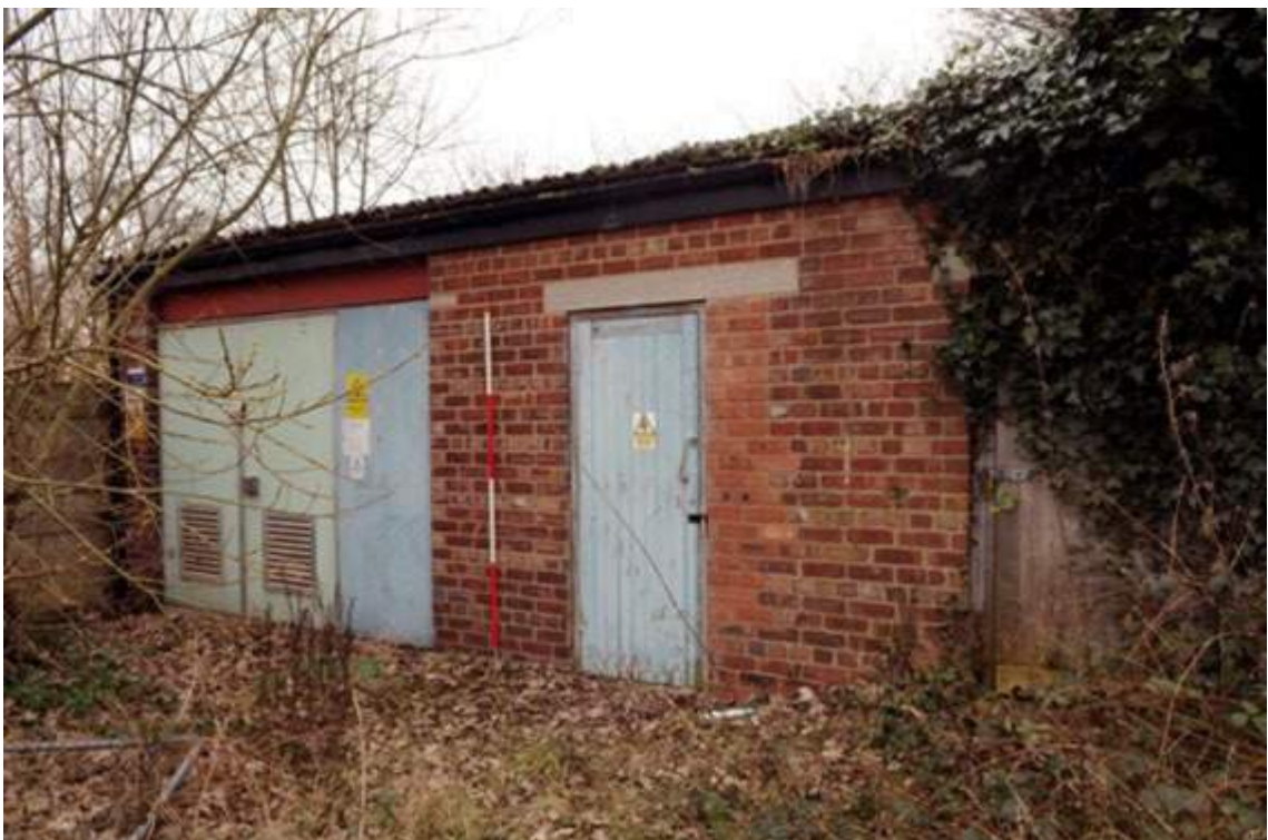
Plate 69. Structure E, north-west elevation (facing south-east)
