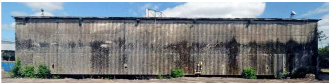
Plate 84. Structure J, west elevation, (facing east)
