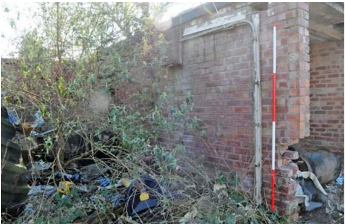
Plate 76. Structure H, west elevation (facing south-west)
