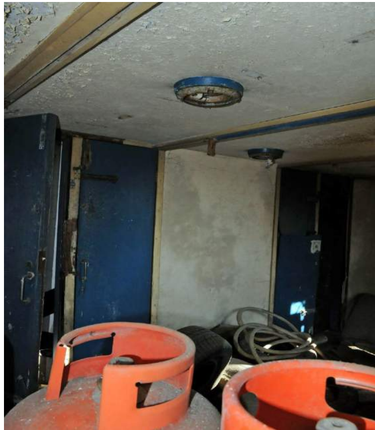
Plate 9. Structure A, east room of the east booth (Facing east)
