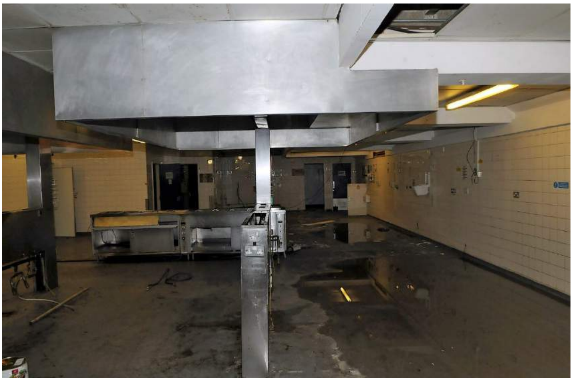
Plate 19. Structure B west end, ground floor kitchen area (facing east)
