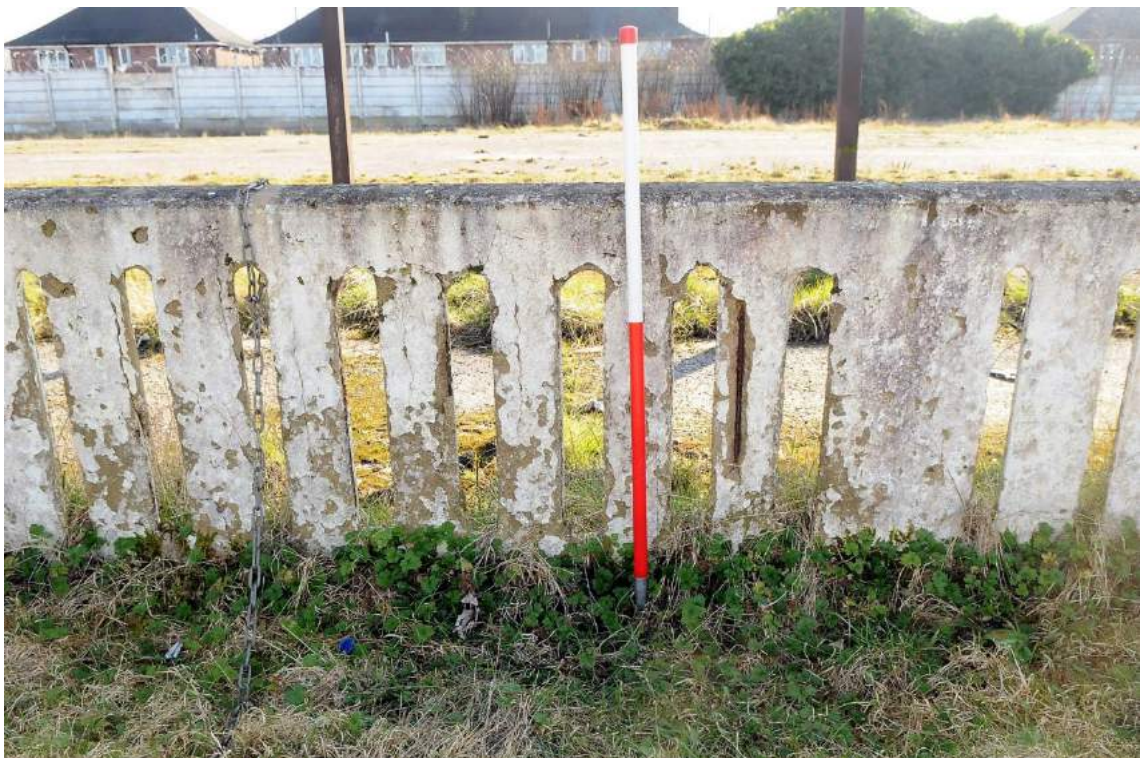
Plate 78. Structure I, inner face of the trackside fence exhibiting a semi-trowelled finish (facing south)
