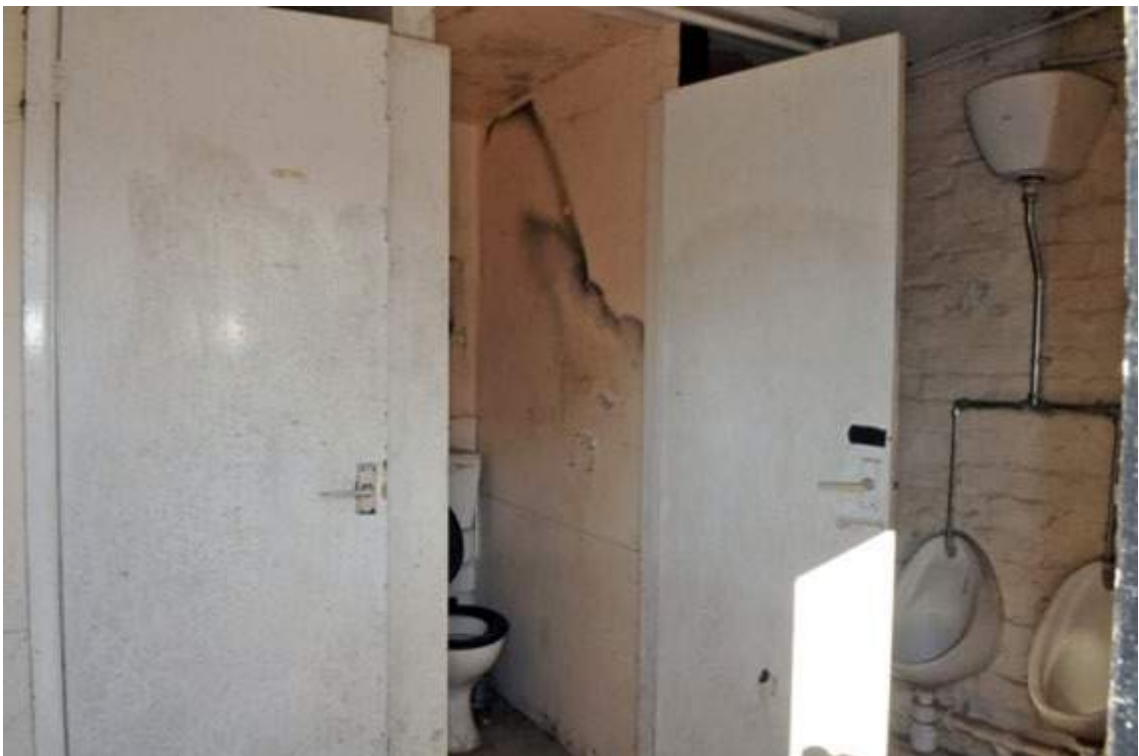
Plate 96. Structure L, interior view of WCs (facing north-east)
