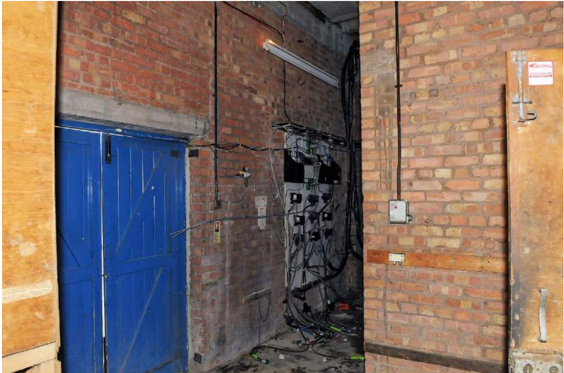
Plate 22. Structure B west end, Phase IV stores to the north of the Phase II section (facing east)
