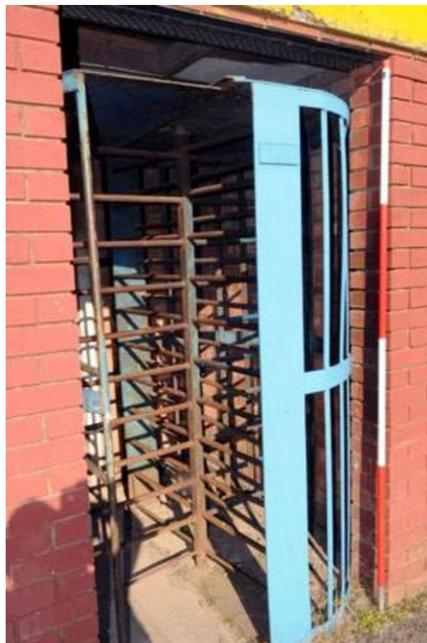
Plate 63. Structure C, Mayor turnstile (facing north)
