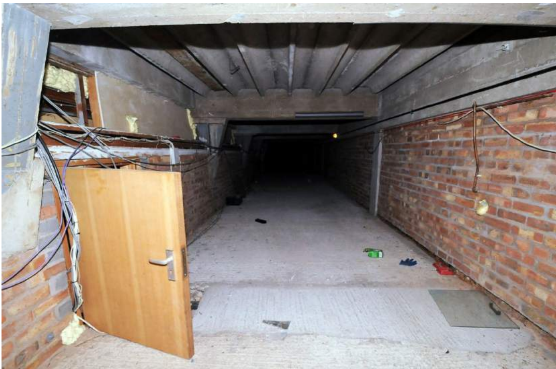
Plate 55. Structure B, Bison Beam and block floor in the void next to the kitchen
