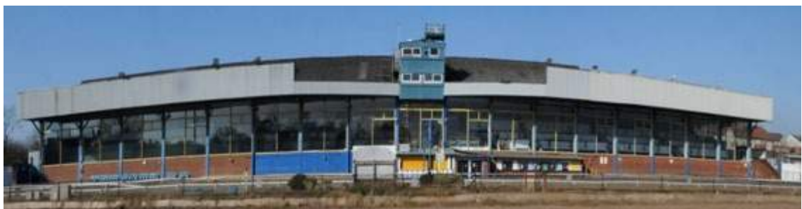
Plate 16. Structure B, south elevation (facing north)
