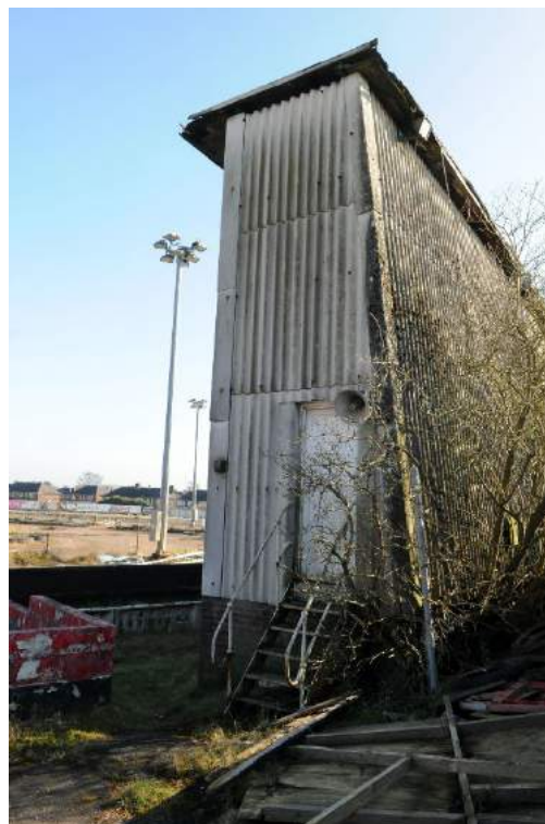
Plate 85. Structure J, north elevation (facing south)
