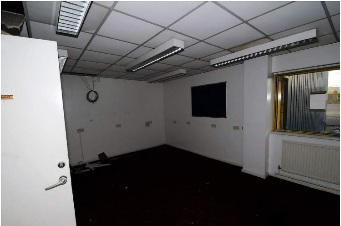
Plate 40. Structure B east end, Operations Manager's office (facing north-west)
