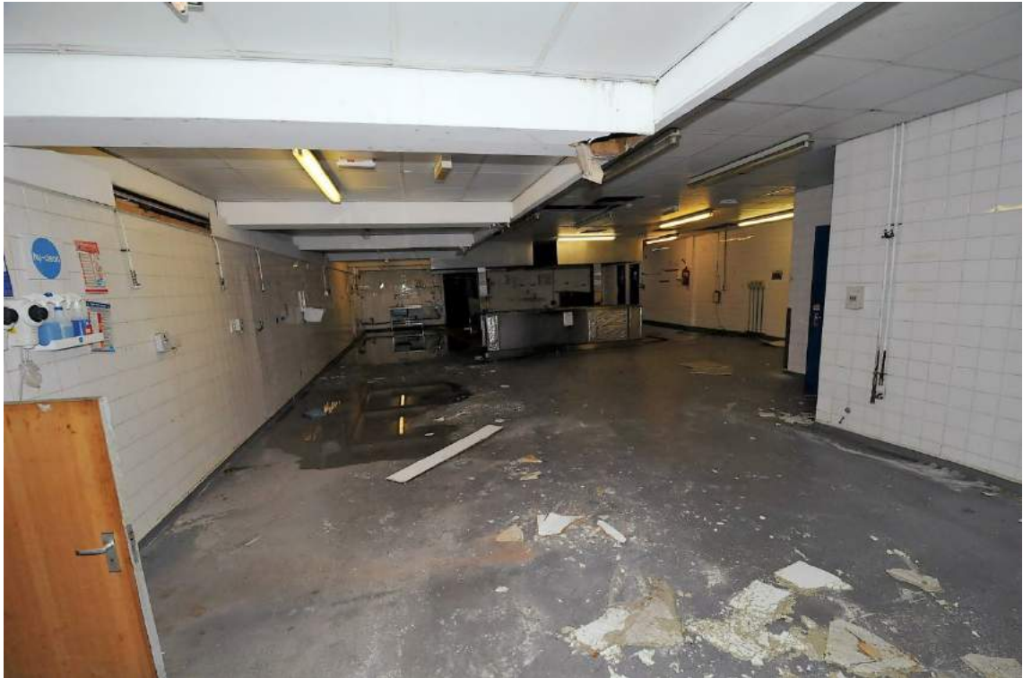
Plate 20. Structure B west end ground floor kitchen area (facing west)
