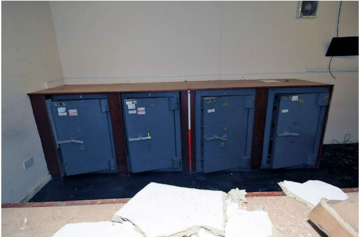
Plate 42. Structure B east end, Chubb safes in cash room
