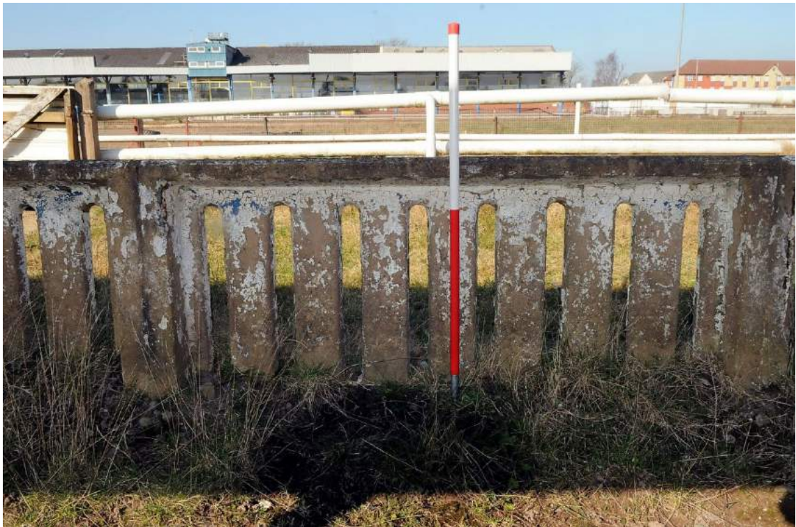
Plate 79. Structure I, outer face of the trackside fence (facing north)
