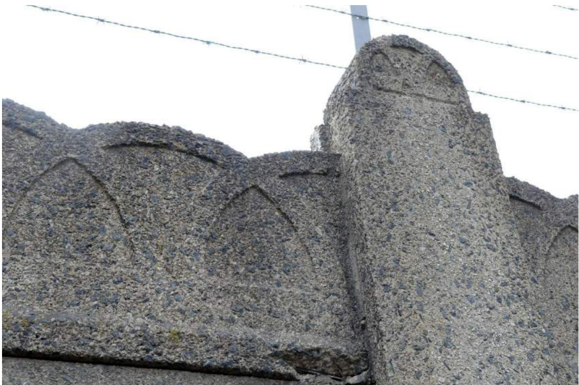
Plate 82. 1950s Perimeter fencing, detail
