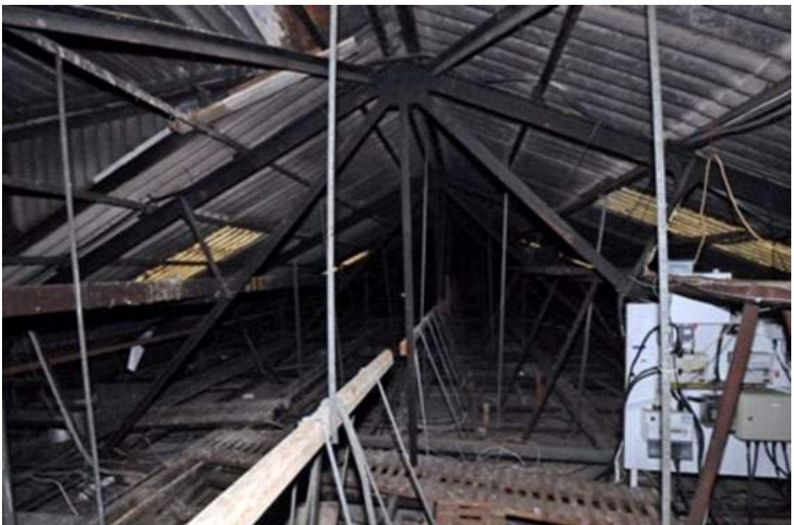
Plate 59. Structure B roof, Phase II roof trusses (facing east)
