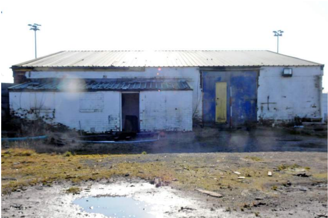
Plate 66. Structure D, north-east elevation (facing south-west)
