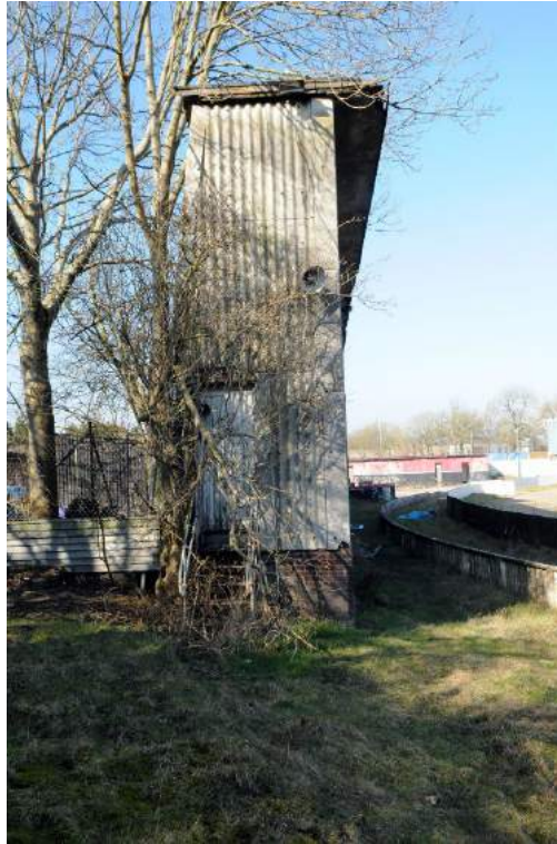
Plate 86. Structure J, south elevation (facing north)
