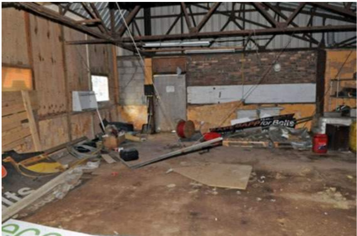
Plate 67. Structure D, interior aspect (facing south-west)
