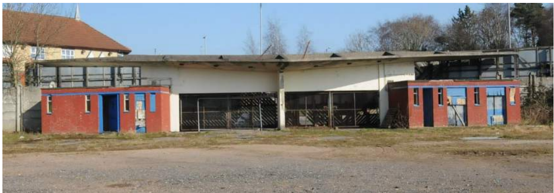
Plate 2. The main entrance (Structure A), south-west elevation showing the two brick booths and concrete canopy (facing north-east)
