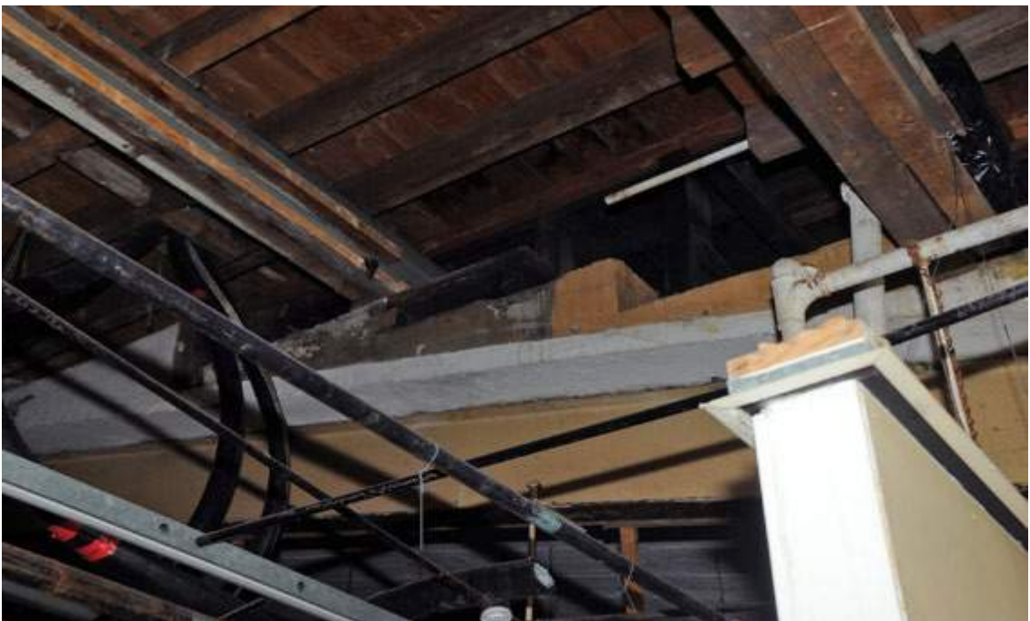
Plate 53. Structure B, the underlying cast in situ terraces of the Phase I stand exposed at the interface with Phase II.
