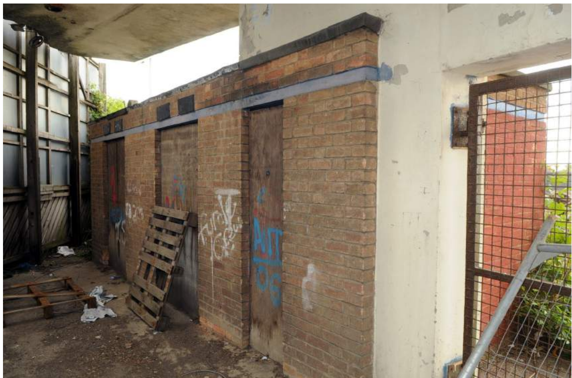
Plate 10. Structure A, north-east elevation of the east booth (Facing south)
