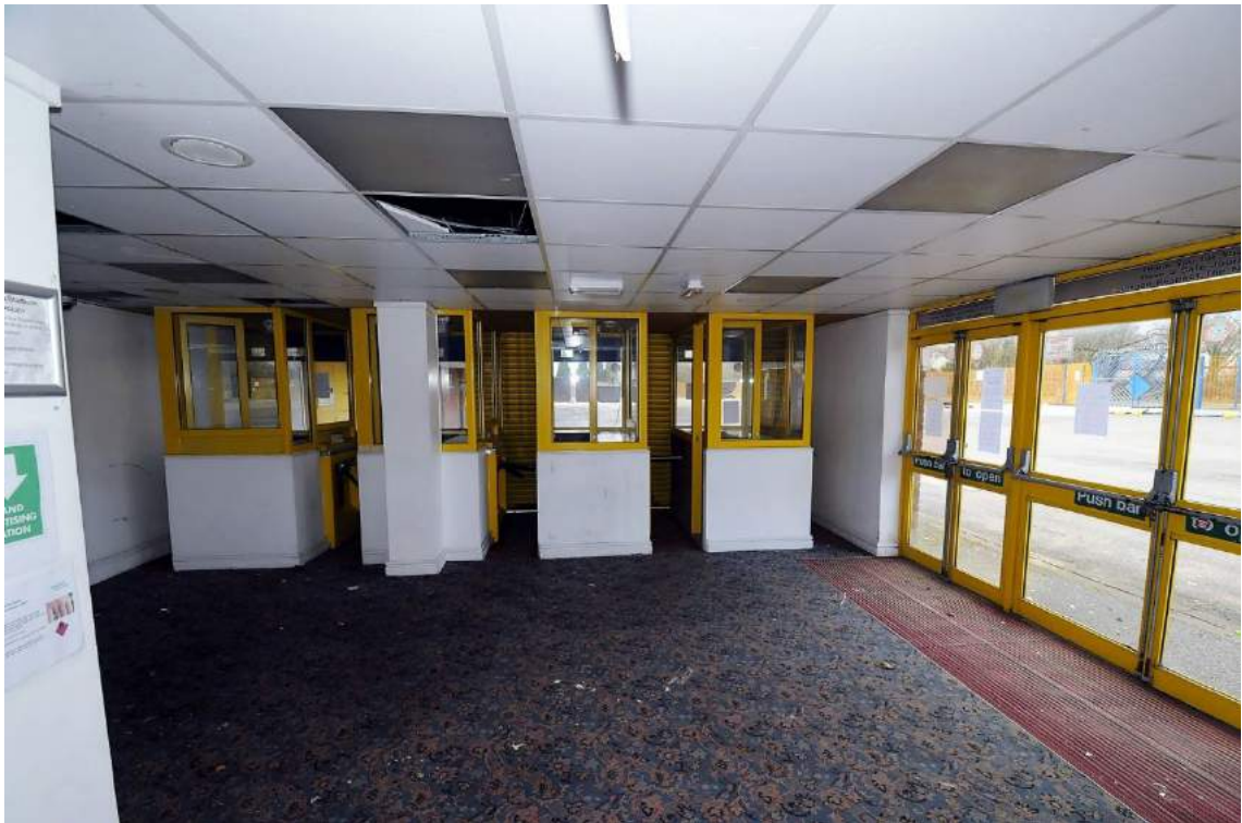
Plate 34. Structure B central, turnstiles (facing west)
