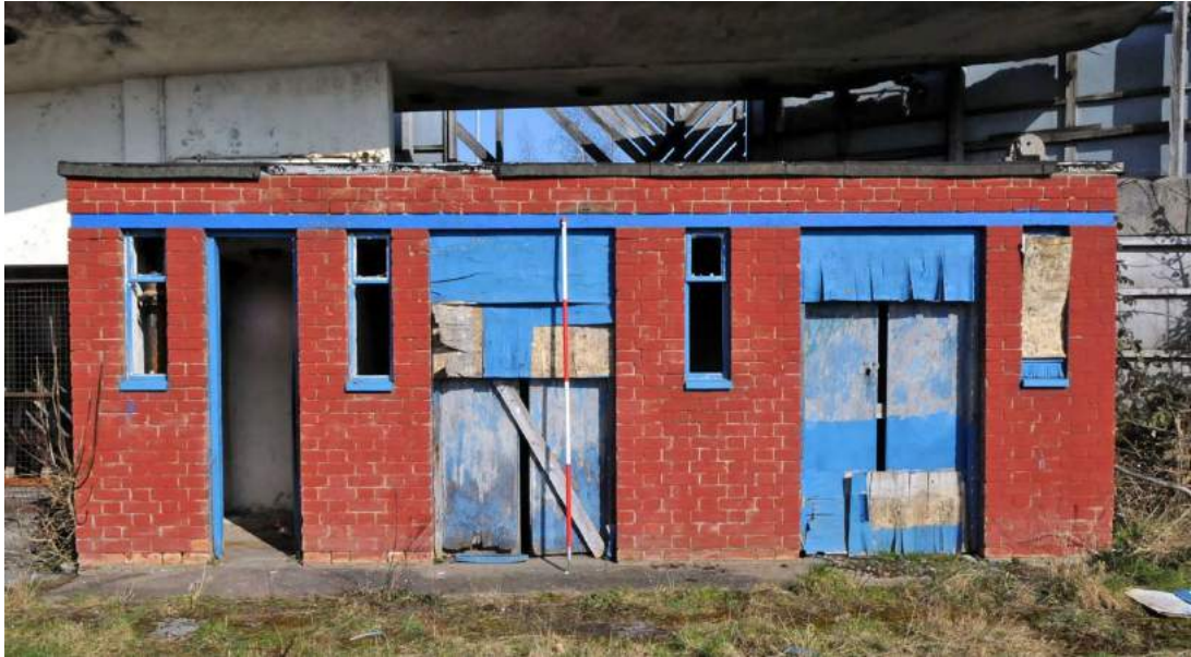
Plate 7. Structure A, south-west elevation of the east booth (facing north-east)
