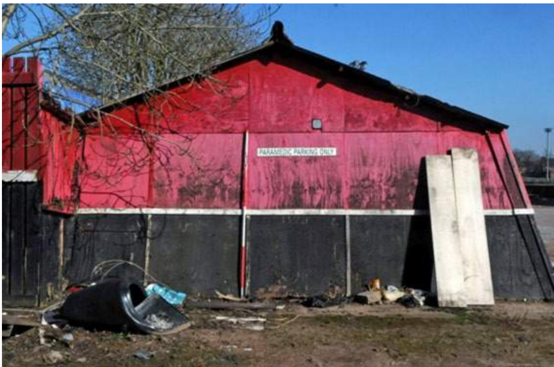
Plate 92. Structure L, possible speedway building, west elevation (facing east)
