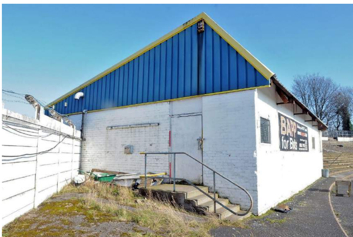
Plate 65. Structure D, north-west elevation (facing north-east)
