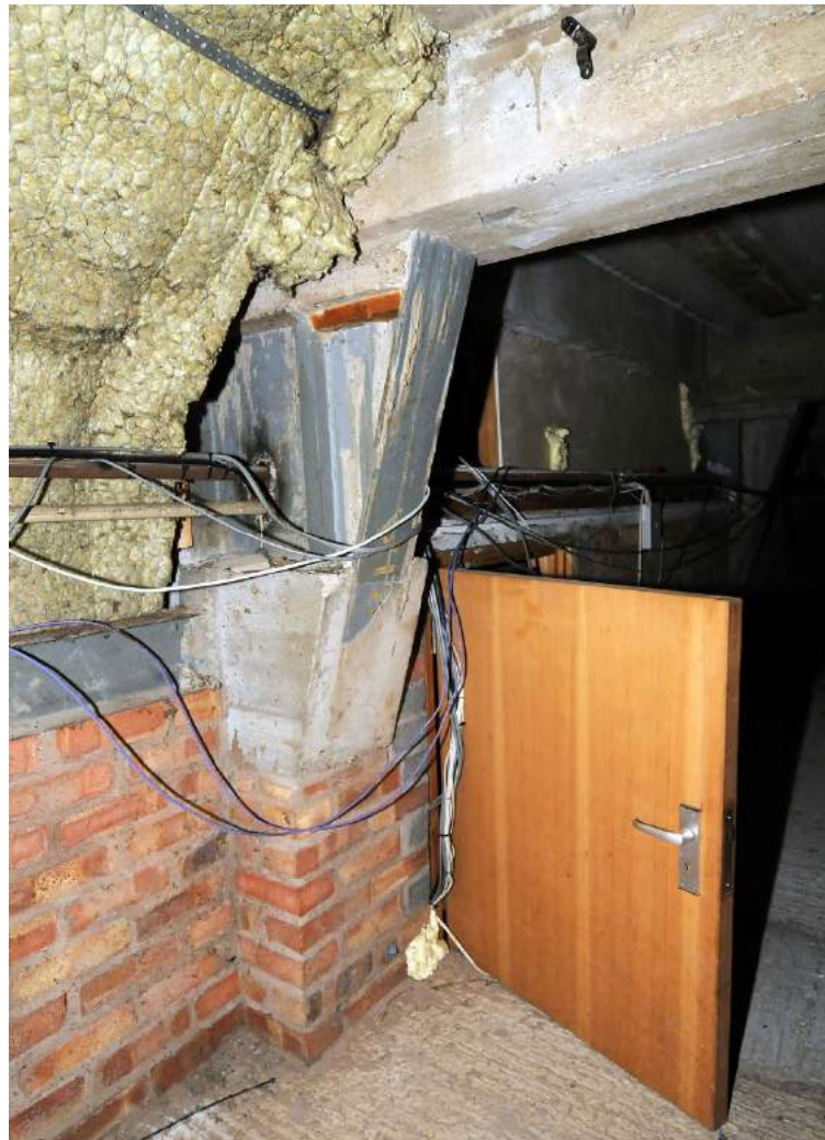
Plate 56. Structure B, detail of main beam and brace supporting the Bison beams.
