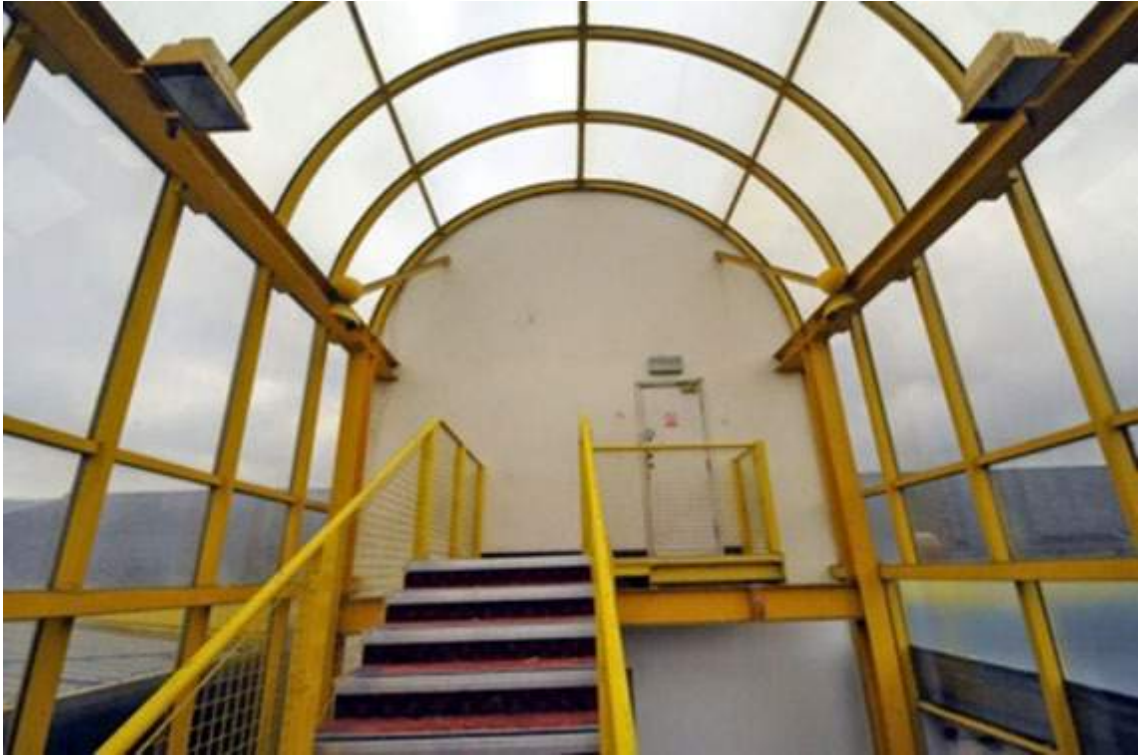
Plate 44. Structure B, second floor landing (facing south)
