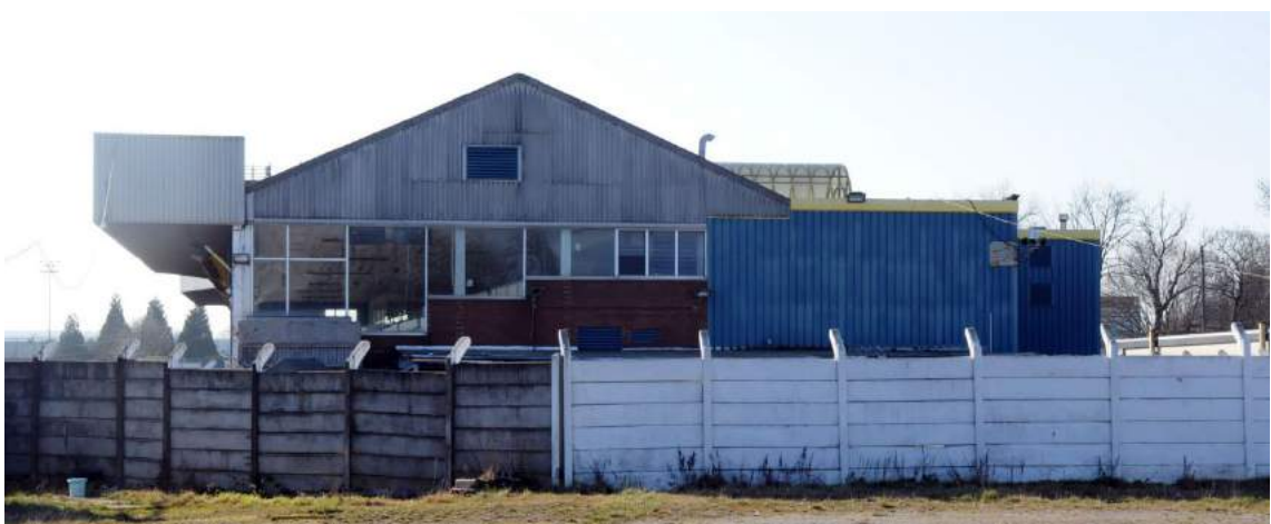
Plate 17. Structure B, east elevation (facing west)
