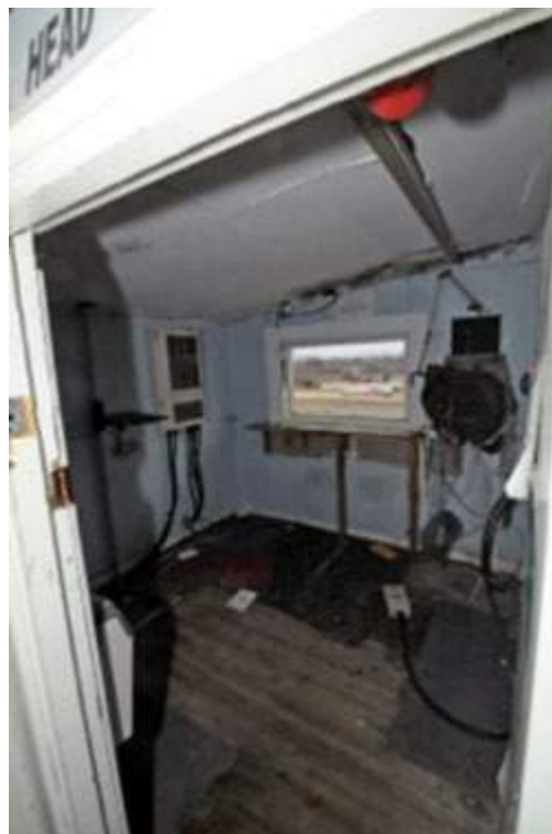
Plate 47. Structure B second floor, hare control room (facing south-east)
