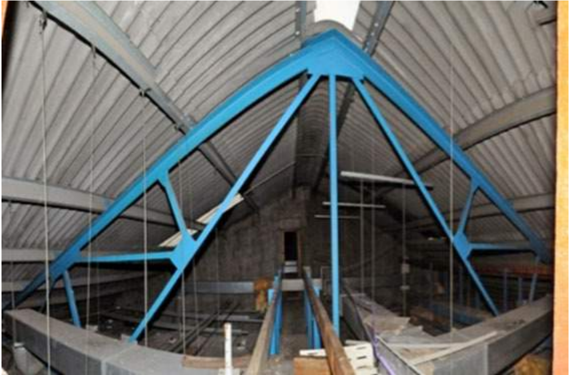
Plate 60. Structure B roof, Phase II roof trusses (facing east)
