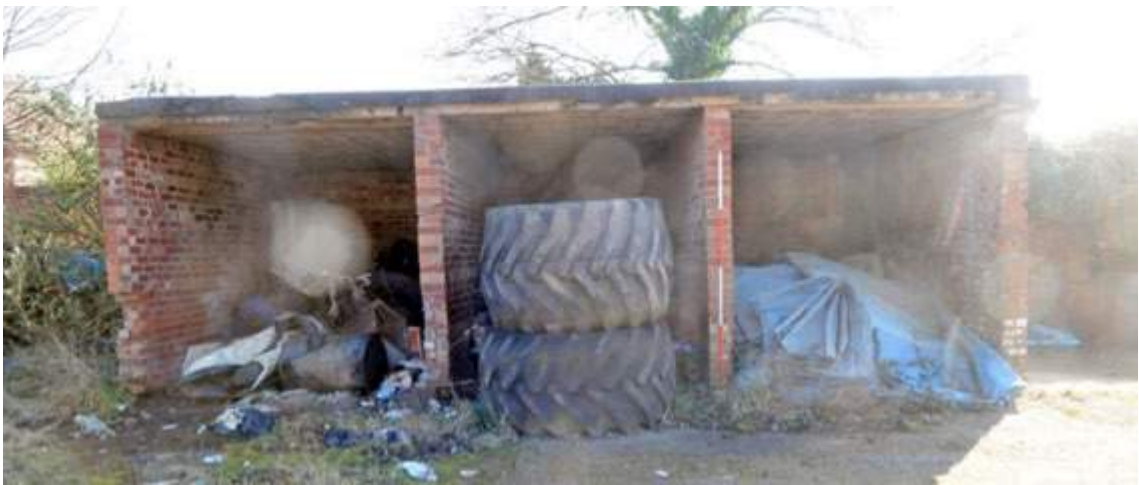
Plate 75. Structure H, north elevation (Facing south)
