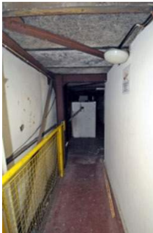
Plate 45. Structure B second floor corridor leading to control and commentary rooms (facing south)
