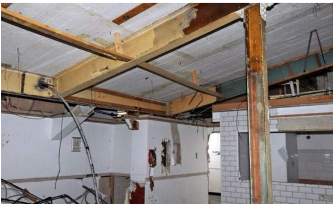
Plate 51. Structure B, ground floor steel frame
