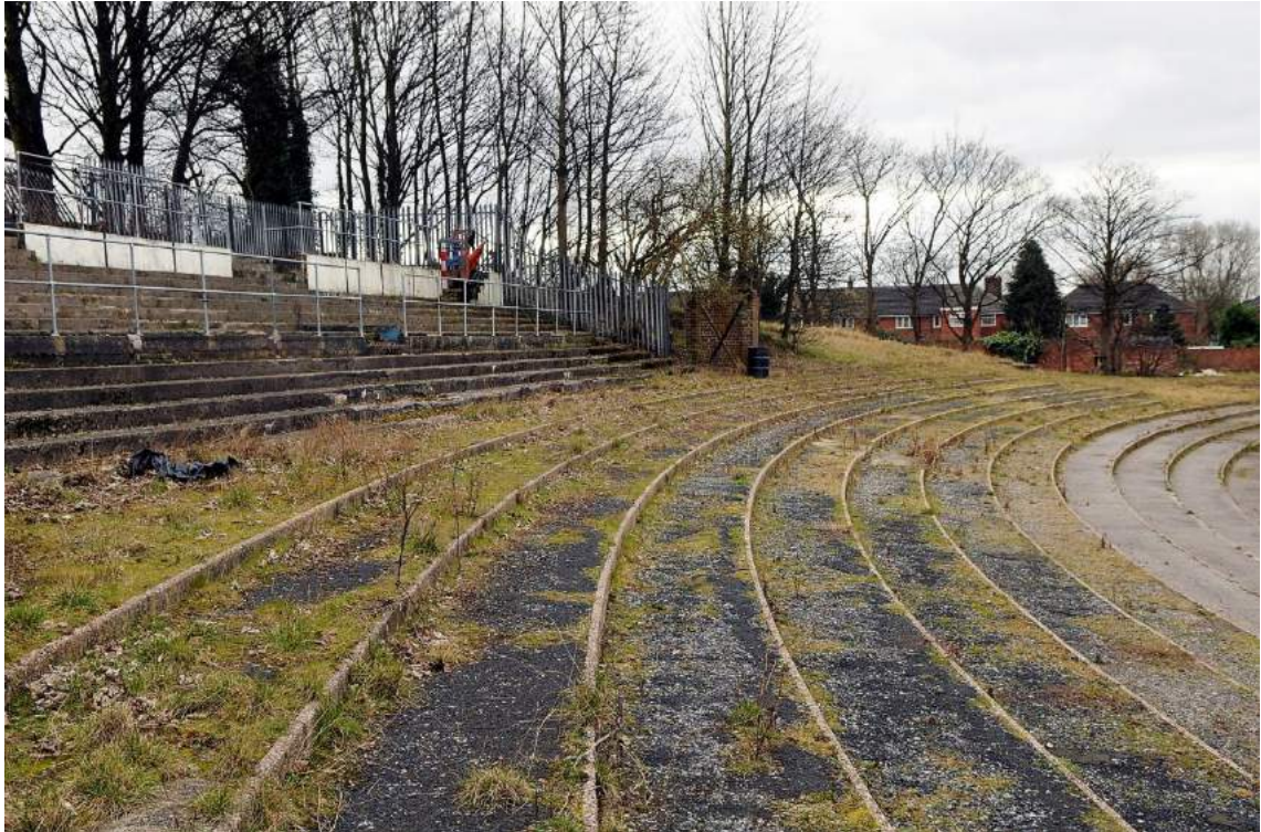
Plate 72. Structure G, The East Stand from the north (facing south)
