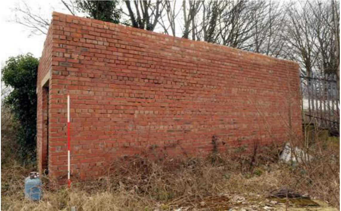
Plate 70. Structure F, west elevation (facing south-east)
