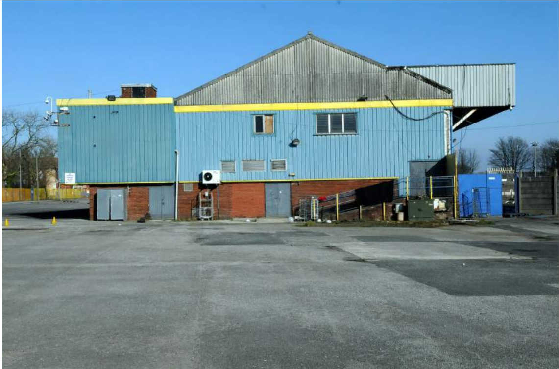
Plate 18. Structure B, west elevation (facing east)
