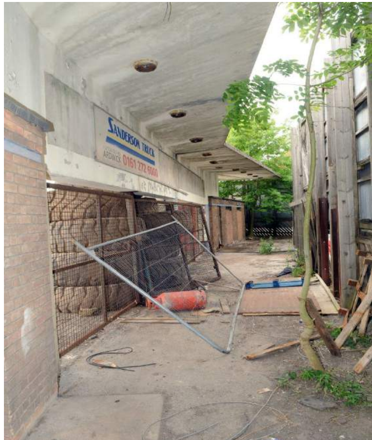
Plate 11. Structure A, canopy at the north side of the entrance (facing north-west)
