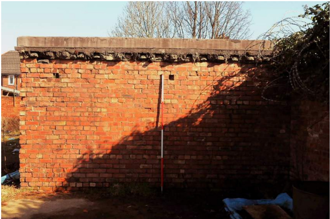
Plate 77. Structure H, east elevation, showing roof construction (facing west)
