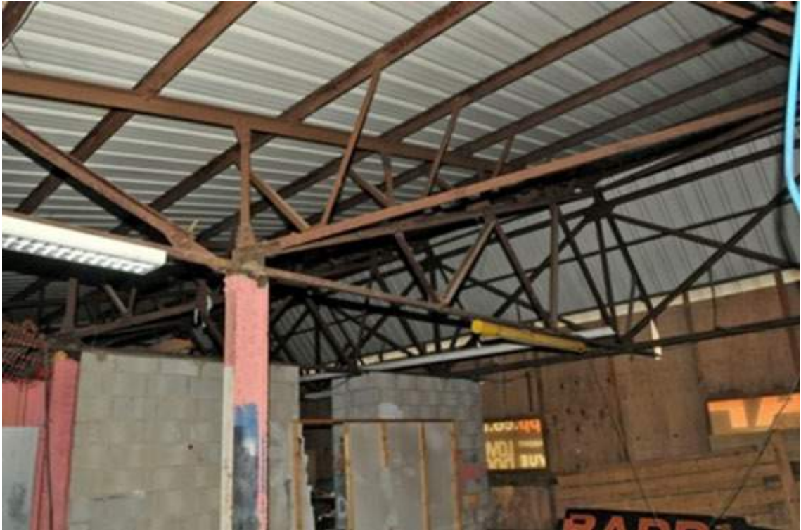
Plate 68. Structure D, example of trusses (facing north-east)
