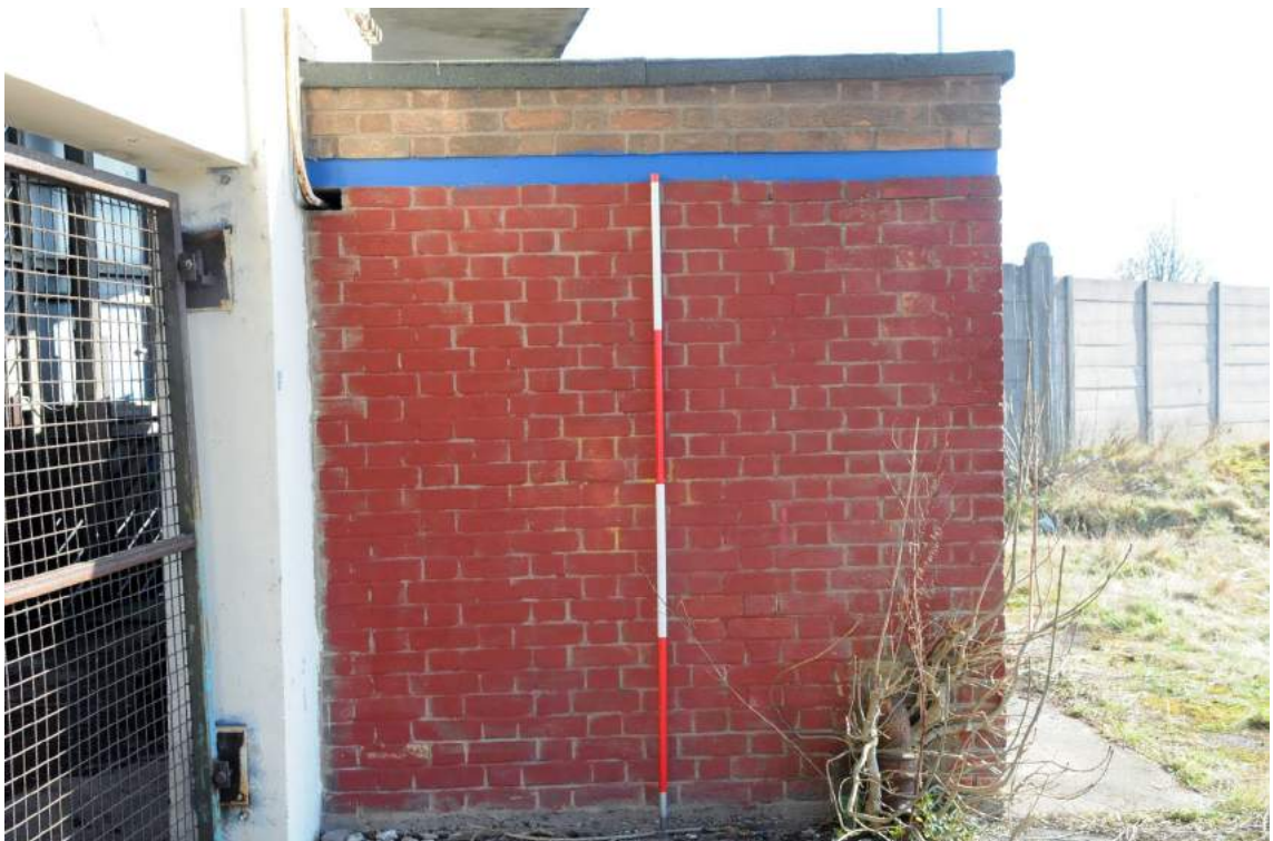
Plate 6. Structure A, south-east elevation of the west booth (facing north-west)
