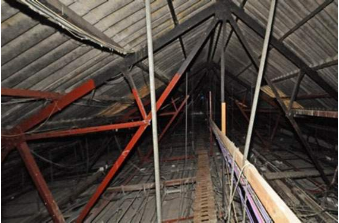
Plate 58. Structure B roof, Phase I roof trusses (facing west)
