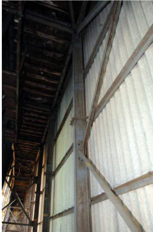
Plate 88. Structure J, internal frame (facing south-west)
