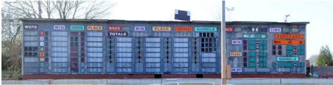
Plate 83. Structure J, east elevation (facing west),
