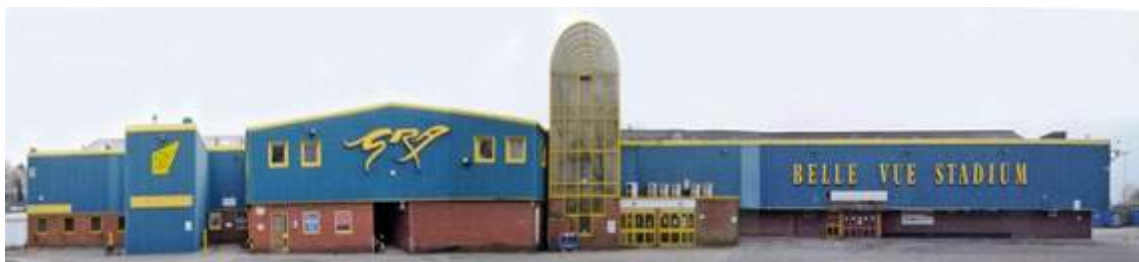
Plate 14. Structure B, north elevation (facing south)
