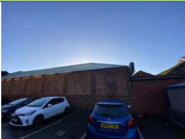
P5: Western end of the northern boundary from Job Centre car park
