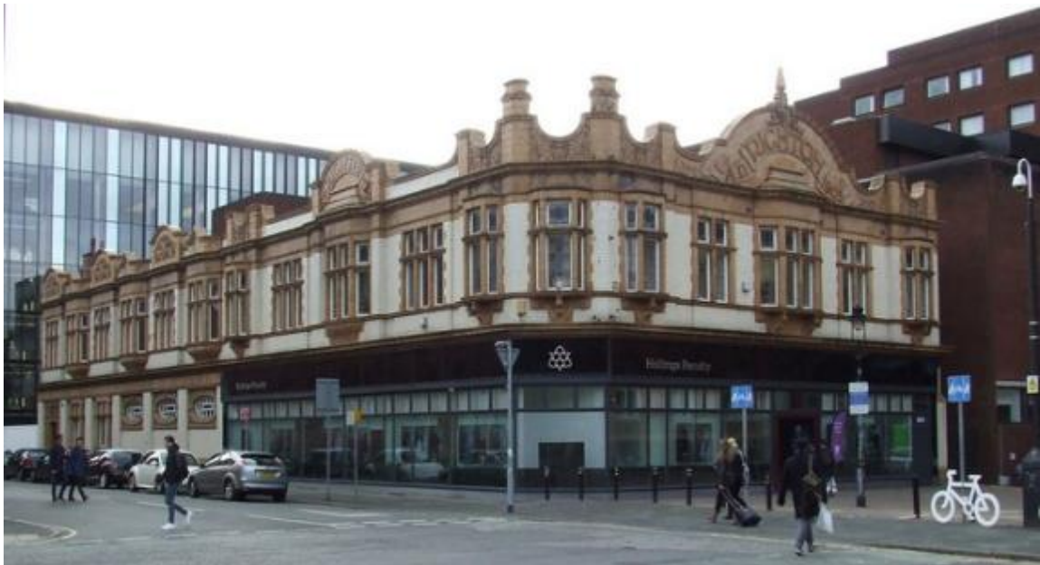
Figure 1: The Righton Building as viewed from Cavendish Street (Source: SLHA 2019).
