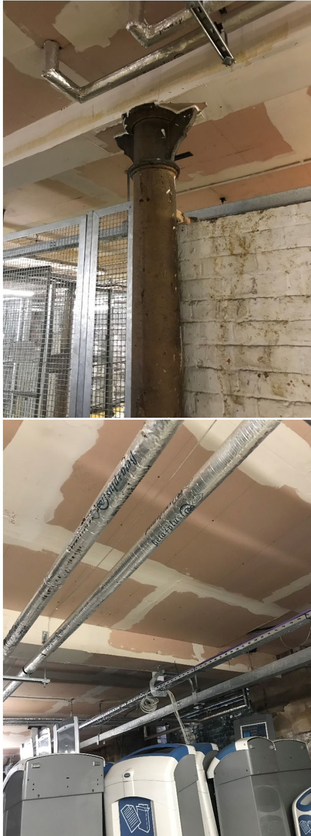
Figure 2 and 3: View of the modern c. 2003 plasterboard under drawing to the ceiling, with detail around the column head and primary structural beam being disguised.
