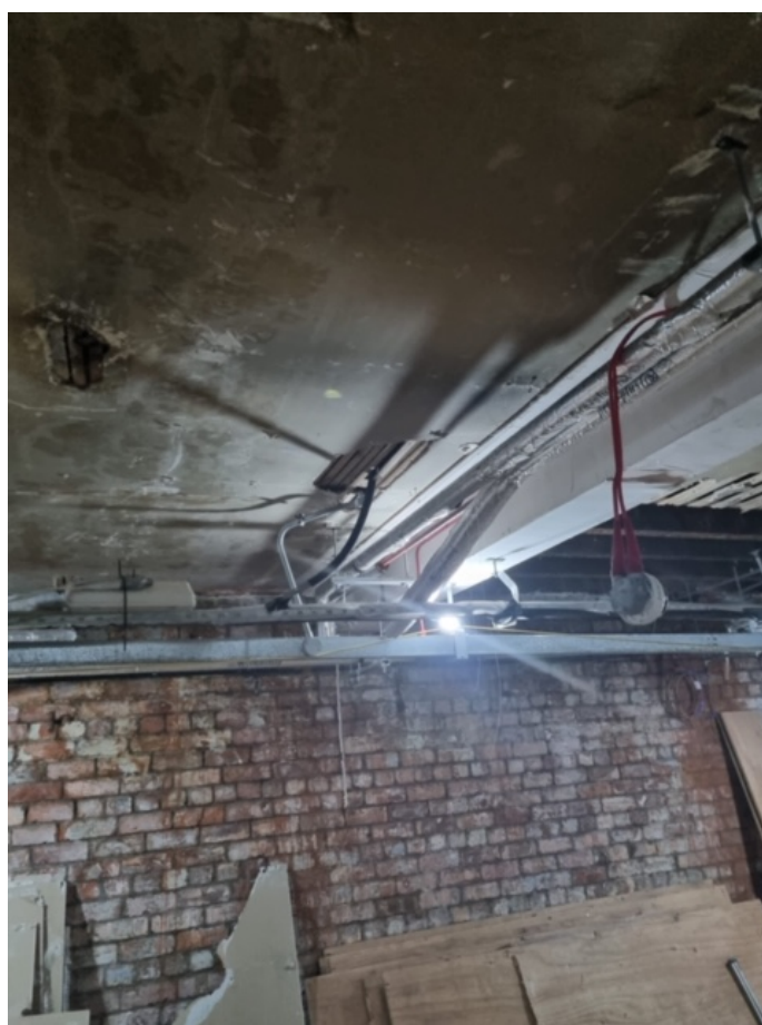
Figure 4 and 5: Views of the surviving lath and plaster ceiling as uncovered in January 2022, not the non-decorative, incomplete nature with a large number of services running through the ceiling.
