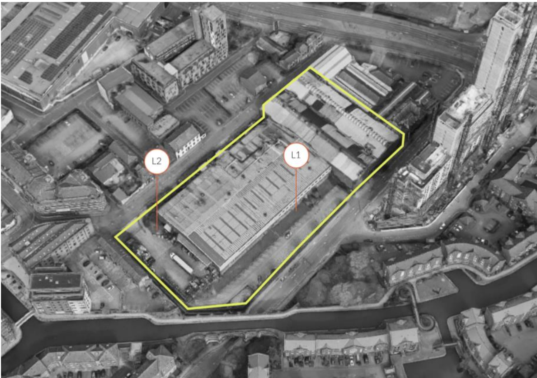
Figure 3 Annotated 3D render image indicating measurement position (courtesy of Google Earth)
