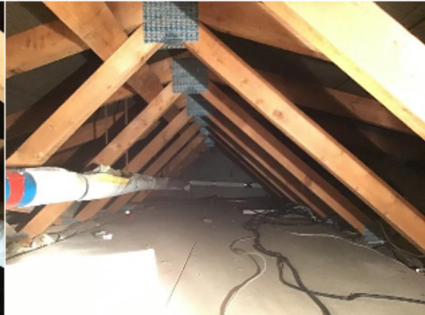
Plate 8: Section 2, roof void
