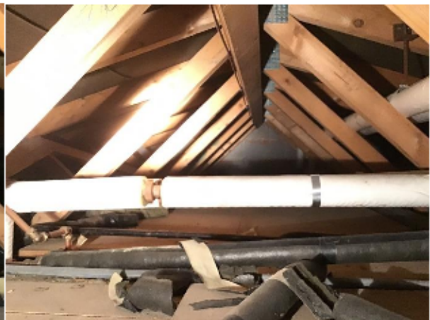
Plate 10: Section 4, roof void
