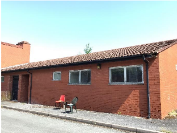
Plate 1: Section 3, from south
