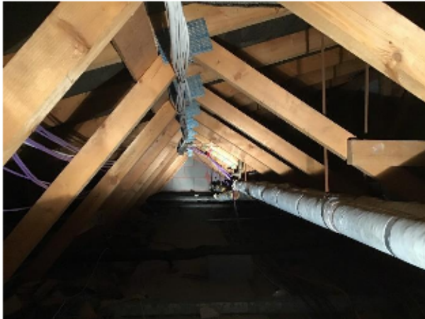
Plate 7: Section 1, roof void
