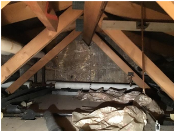
Plate 9: Section 3, roof void
