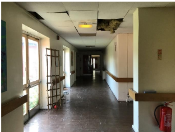
Plate 5: Section 1, main corridor
