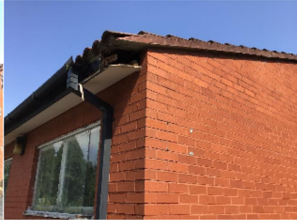
Plate 2: Soffit on Section 3
