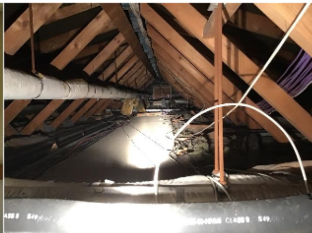
Plate 6: Section 1, roof void
