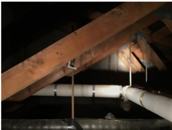
Plate 11: Section 5, roof void
