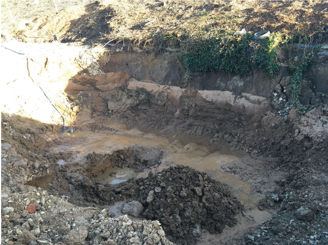
Plate No. 1: Fuel Tank Excavation
