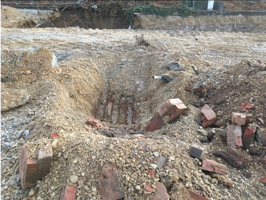
Plate No. 1: VAL01 Excavation
