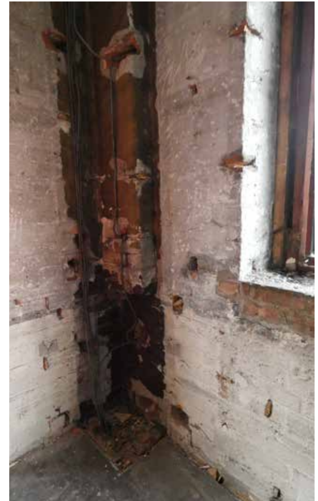
3.51 Flue, S002, Second Floor
