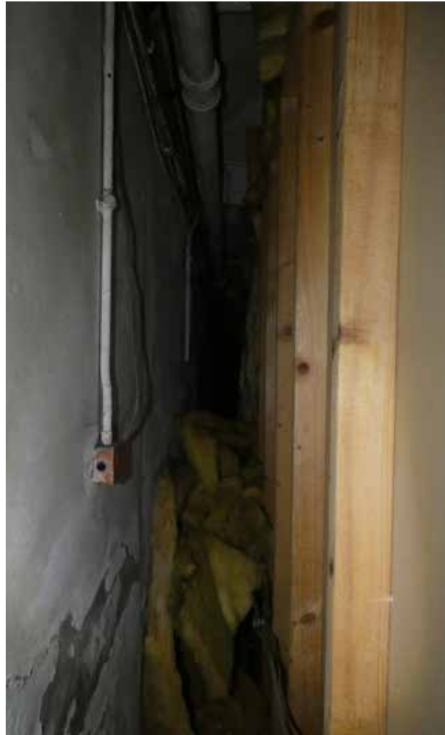
3.15 Basement, view behind B019-21 (Install)
