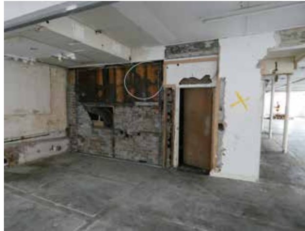
3.45 Partitions and screen around timber staircase, First Floor
