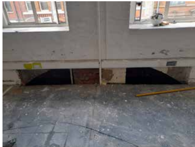
3.46 Arch revealed in front wall to Newton Street, First Floor
