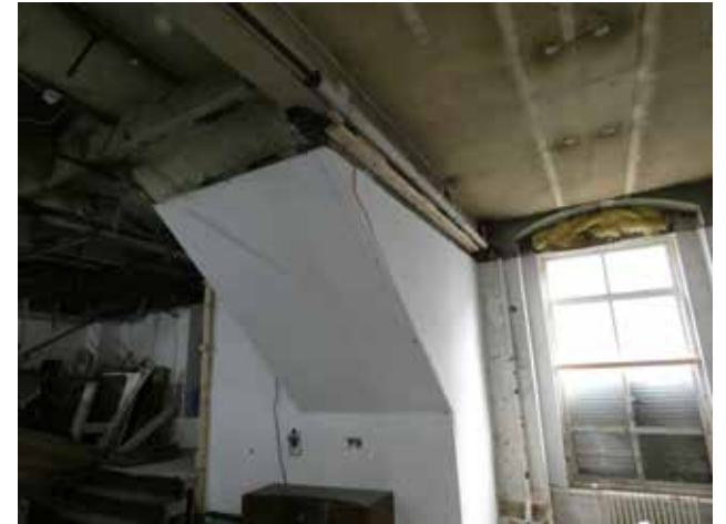
3.42 Plasterboard around timber staircase, Ground Floor
