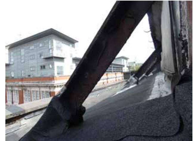
3.104 View of cast iron principle rafters, NW
