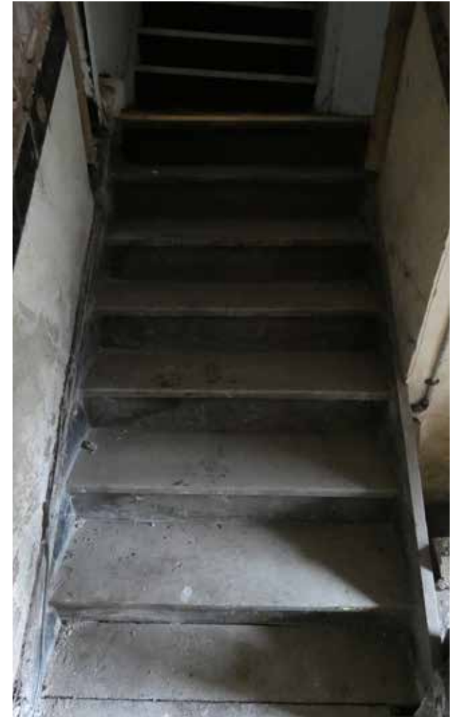
3.37 Ground Floor Stair to Yard
