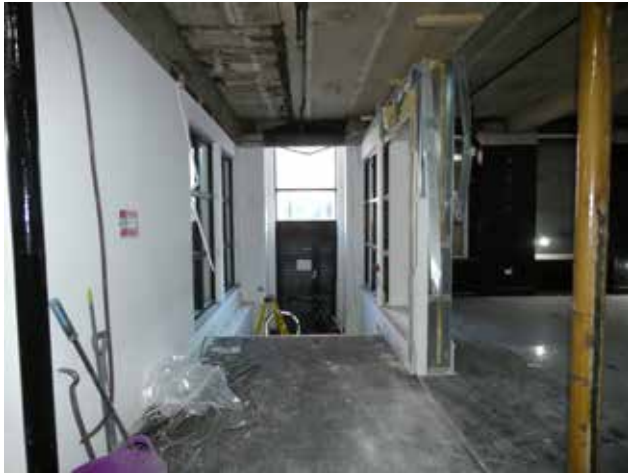
3.35 Partitions forming office - G002, Ground Floor
