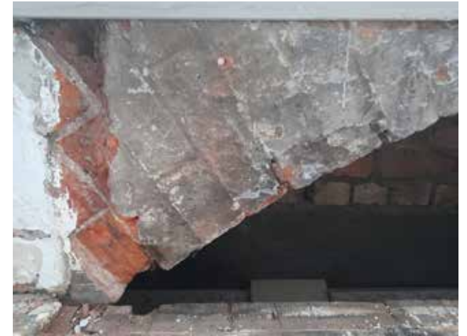
3.47 Arch revealed in front wall to Newton Street, First Floor
