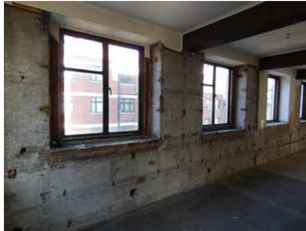
3.53 Part-plastered walls, S002, Second Floor
