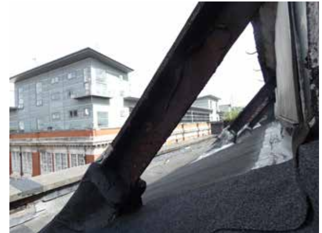
3.6 View of roof with cast iron rafters (Insal)
