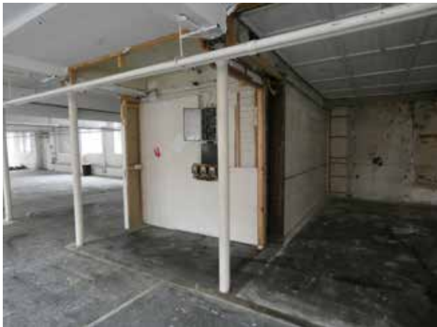
3.44 Partitions around timber staircase, First Floor
