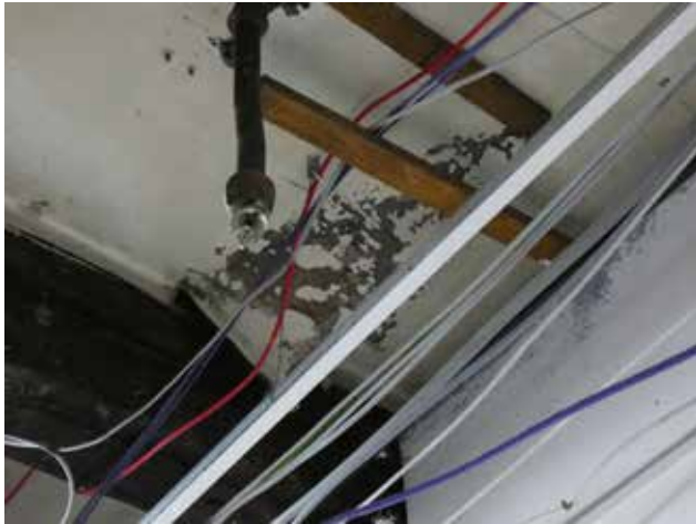
3.39 Ceiling in G001, Ground Floor
