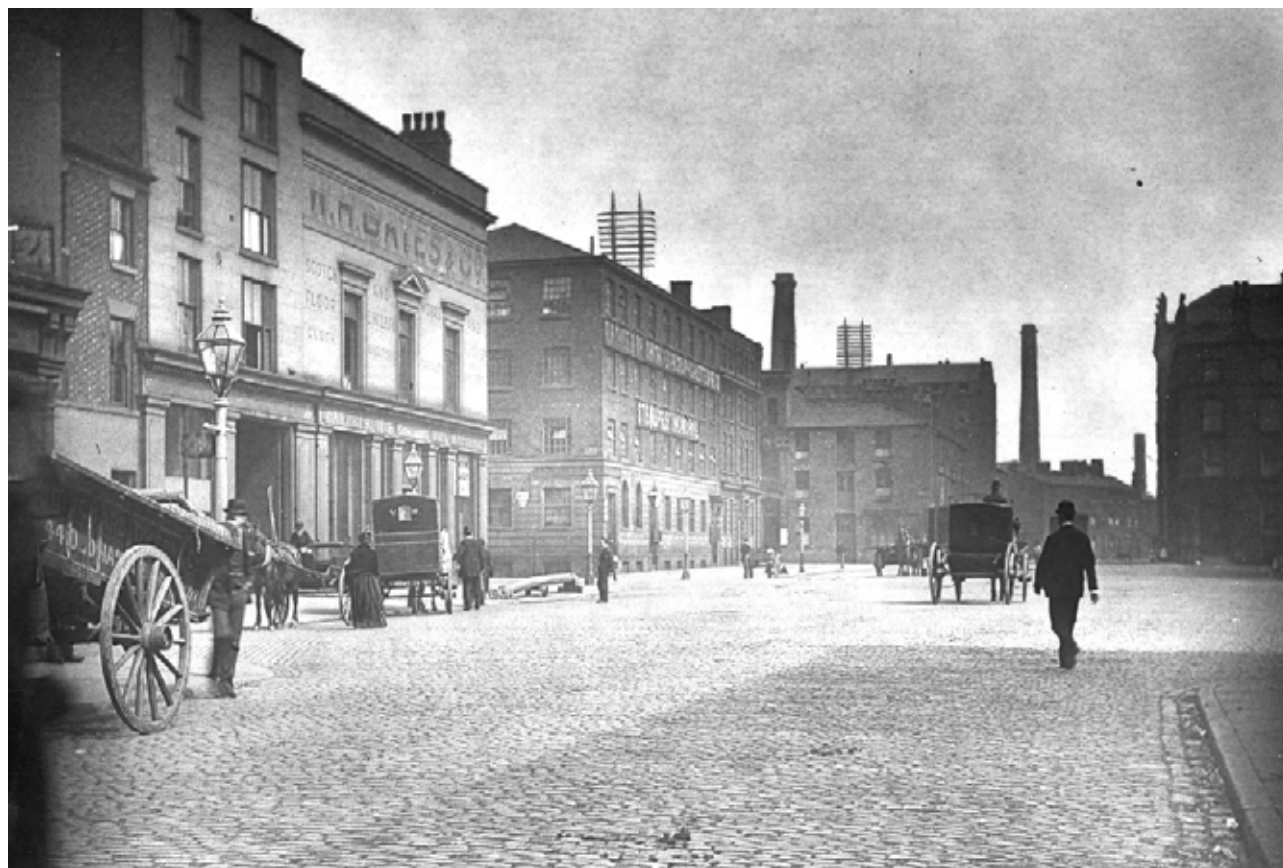
2.15 Stevenson Square looking to Hilton Street, 1891. Manchester Libraries
