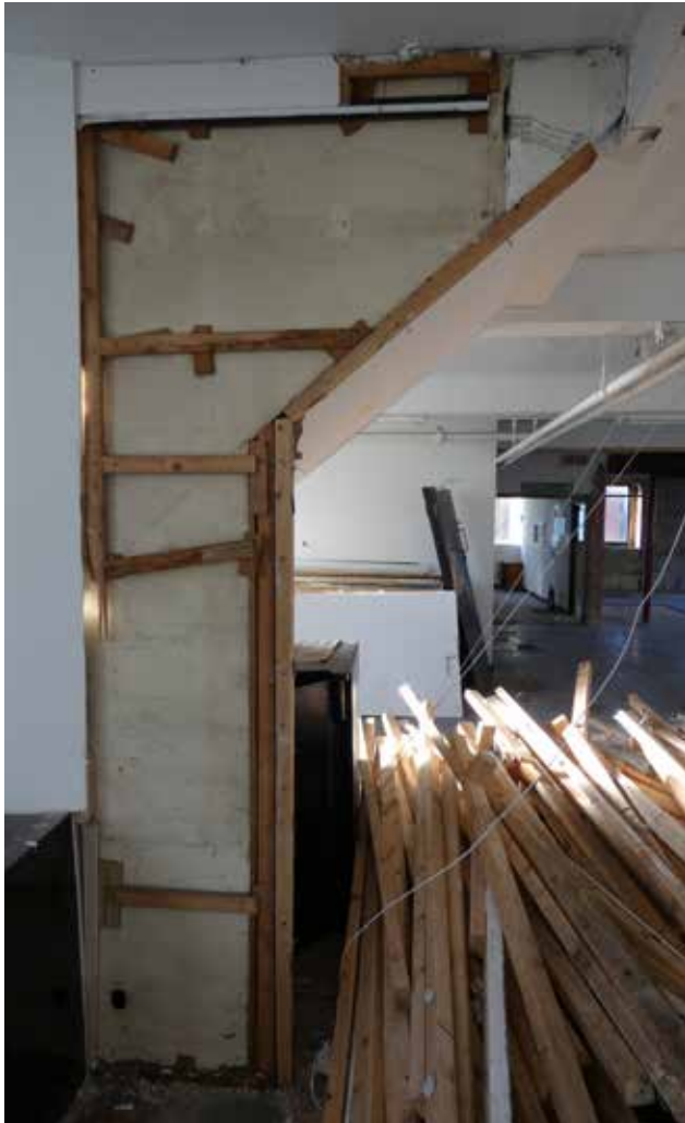
3.52 Partition around timber stair, S002, Second Floor
